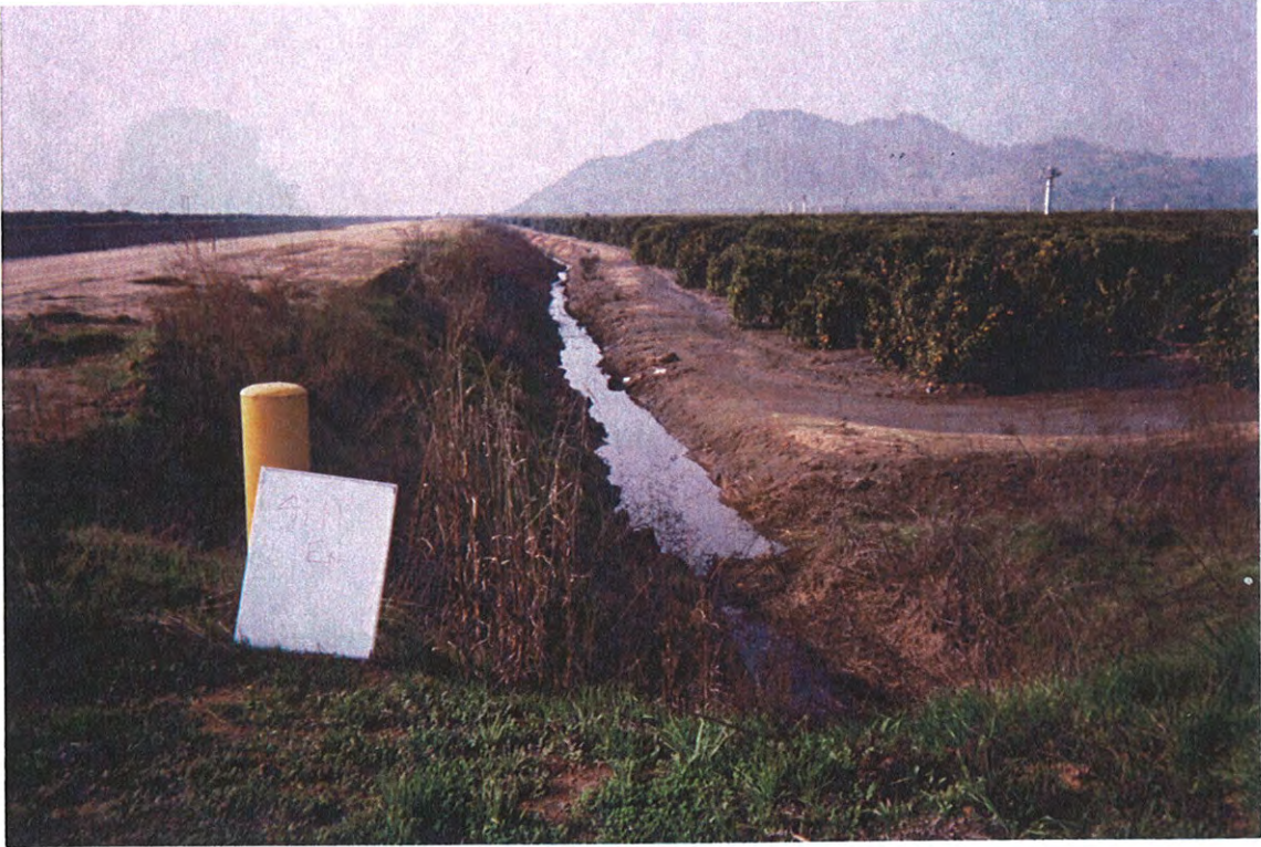
Upstream (eastside looking north)
