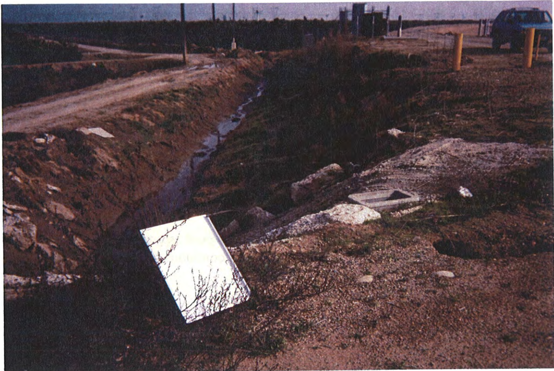
Upstream (looking south)
