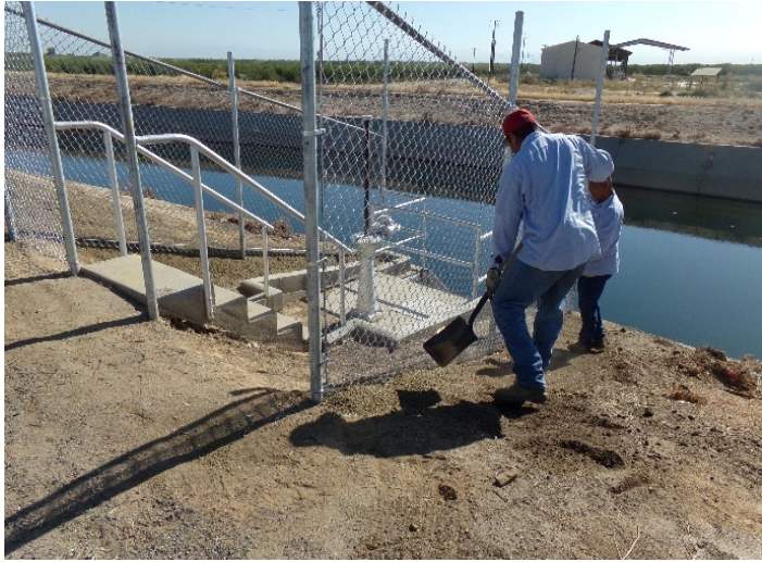
Delano maintenance staff continues embankment maintenance
