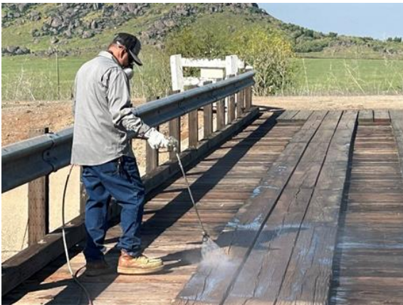
Lindsay maintenance staff performed a deep cleaning and a thorough inspection of all wooden farm bridges and crossings,
