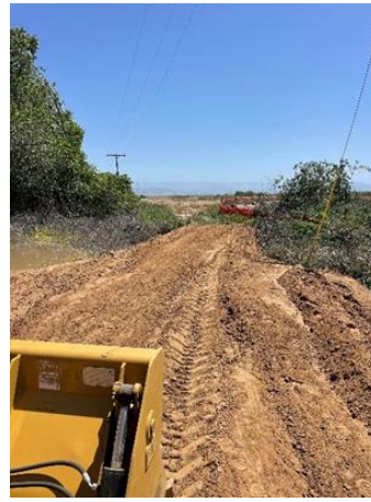
Lindsay maintenance staff made safety precautions to ensure stability near highline pole and addressed the leak causing destabilization at DCTRA pit.
