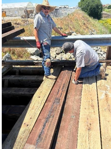
Lindsay maintenance staff began replacing deck boards on the bridge at cottonwood creek.
