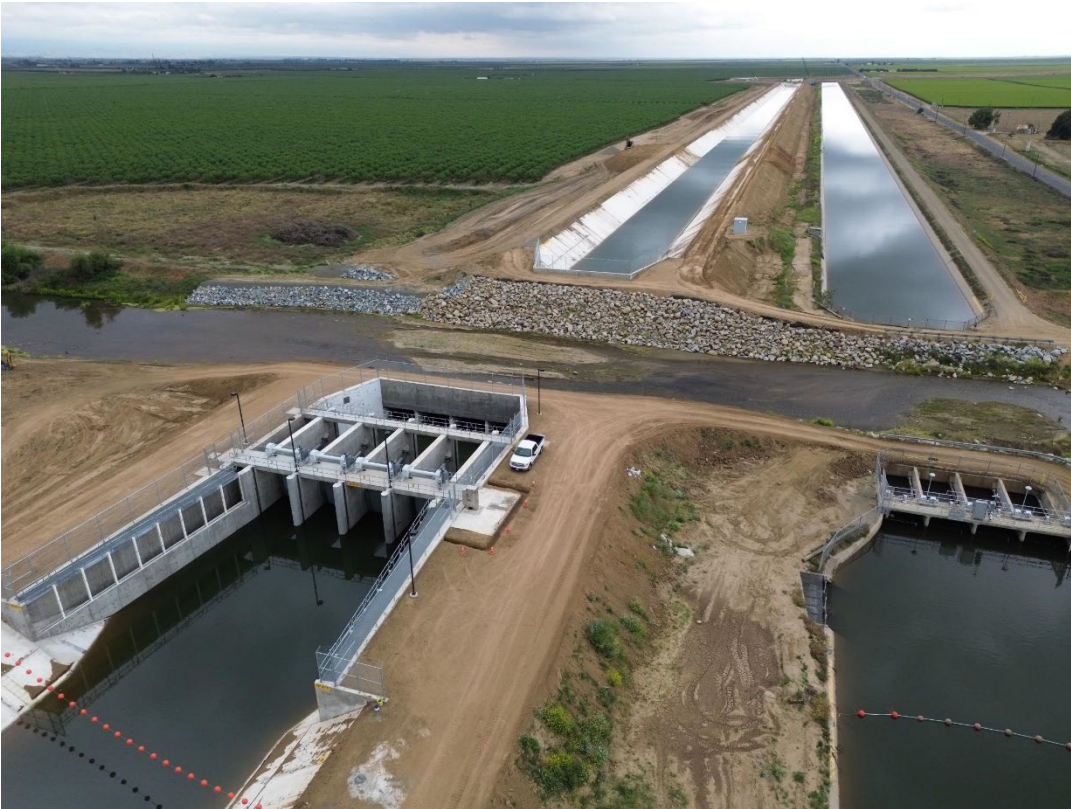
Pre-commissioning at Deer Creek check.
