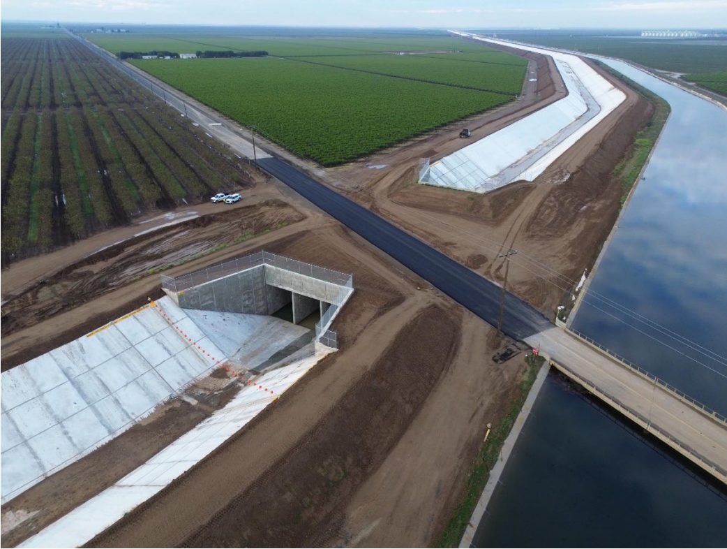
Road 208 Paving was Completed.
