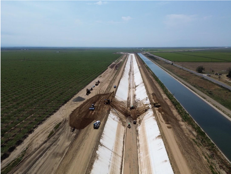
Northern Temporary Earthen Plug was Removed.
