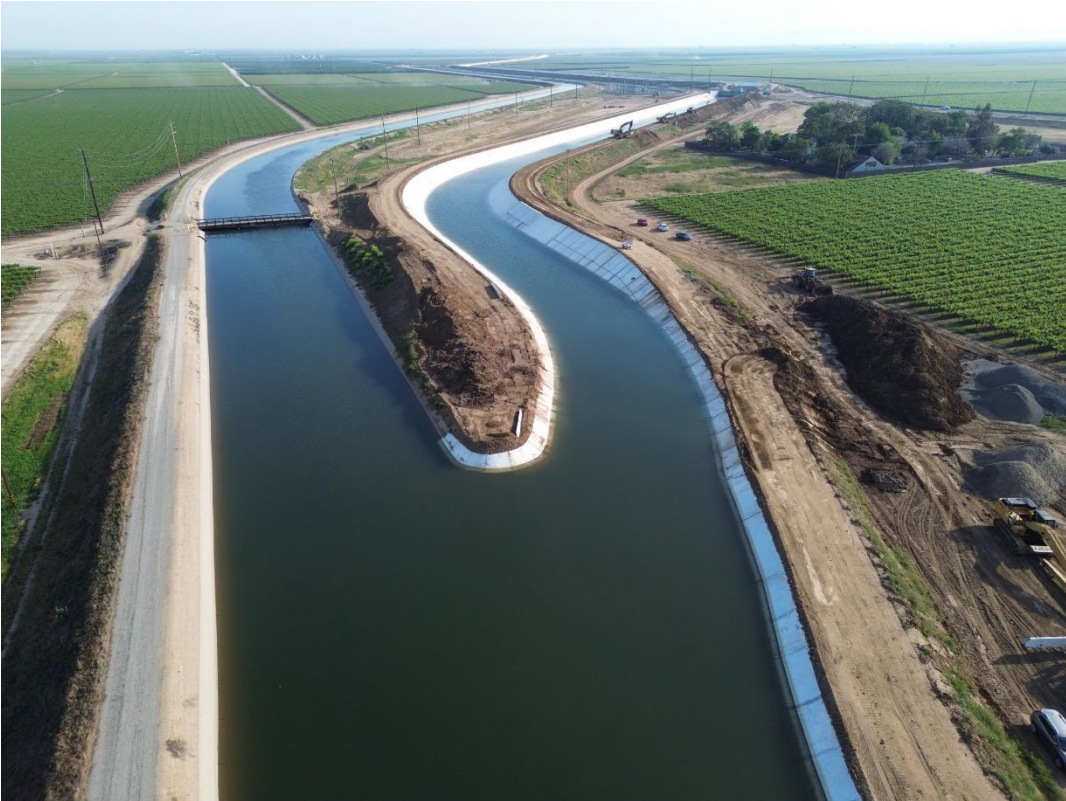
South Tie-in After Earthen Plug Removal.
