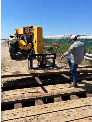
Lindsay maintenance staff began replacing deck boards on the bridge at cottonwood creek.
