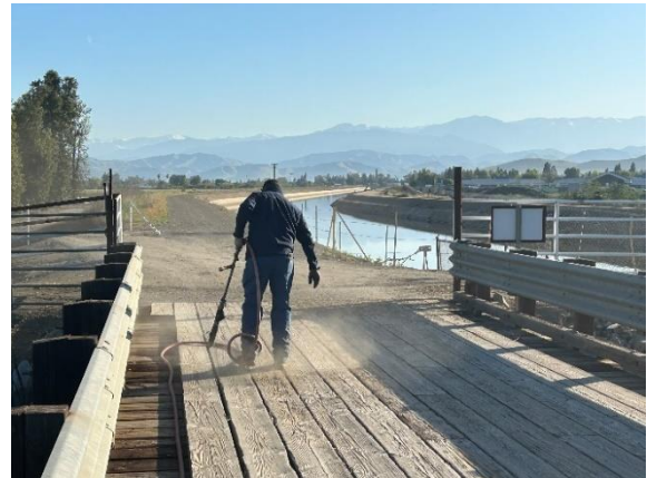
Lindsay maintenance staff performed a deep cleaning and a thorough inspection of all wooden farm bridges and crossings,
