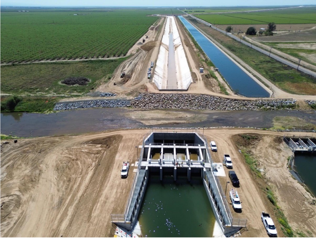
First Canal Fill Between Deer Creek and South Tie-in.
