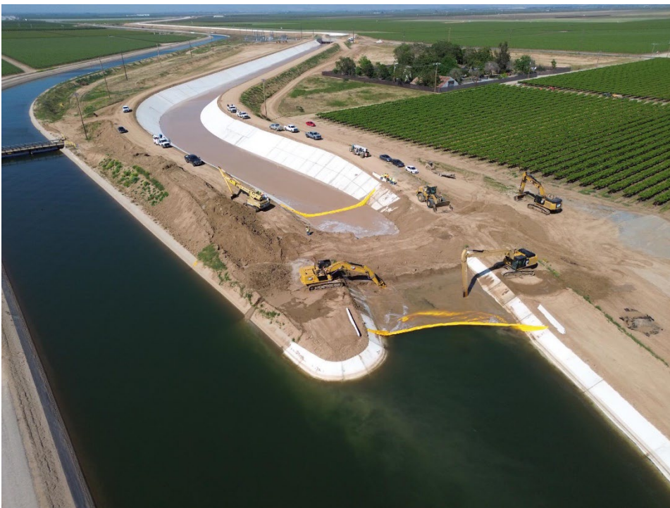
Start of Southern Tie-in Temporary Earthen Plug Removal. Final Breach Conducted after Water Equalized.
