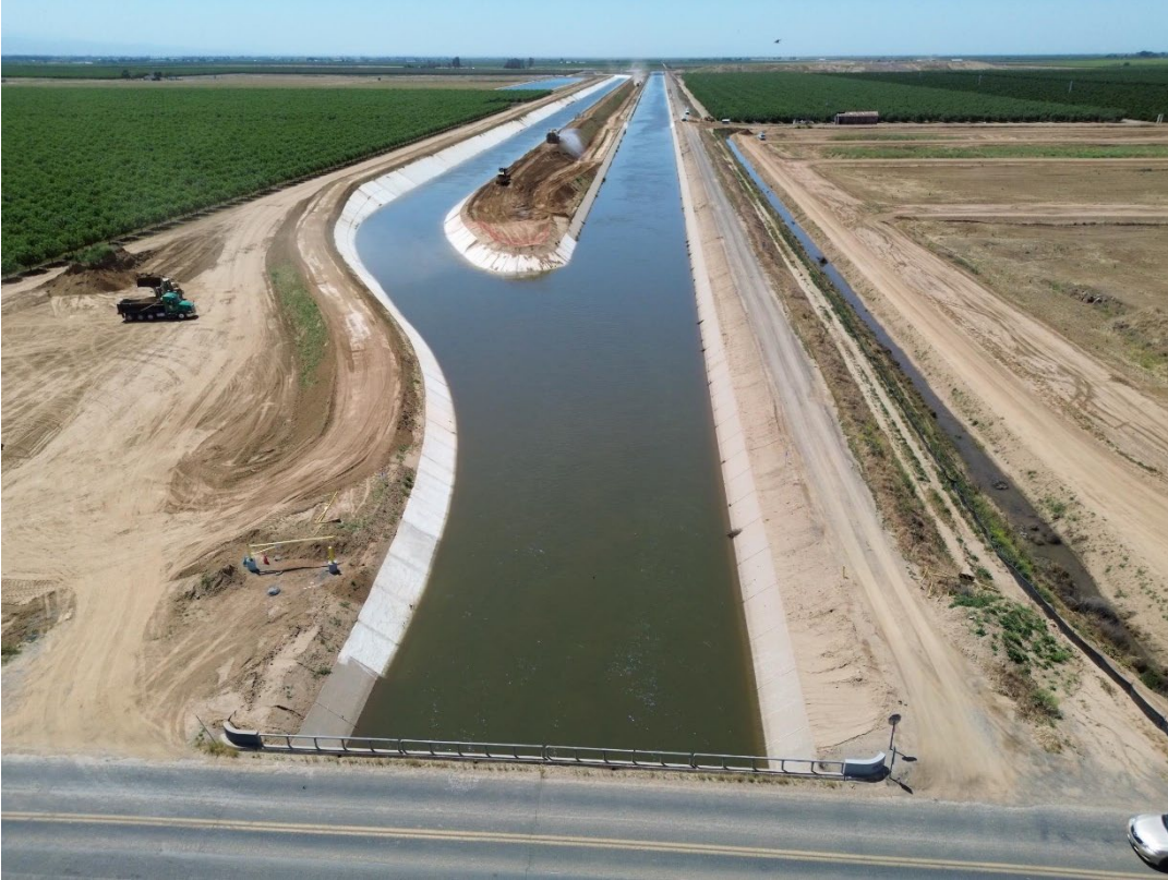
Canal Embankment Placement Above the Canal Lining at the Northern Bifurcation.
