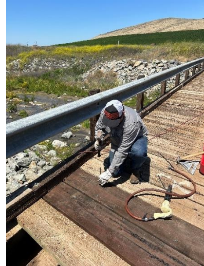
Lindsay maintenance staff began replacing deck boards on the bridge at cottonwood creek.
