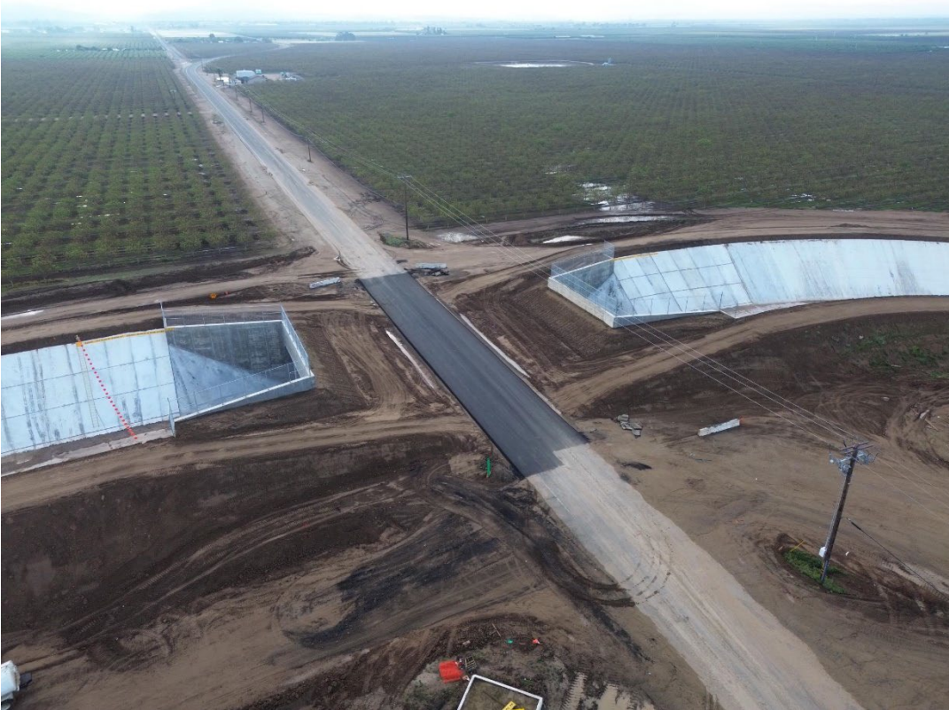
Avenue 95 Road Paving was Completed.
