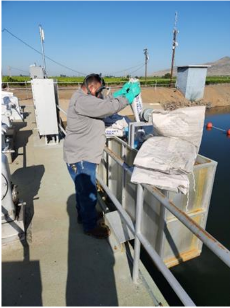
Application of copper sulfate in the canal prism to control algae in the FKC.
