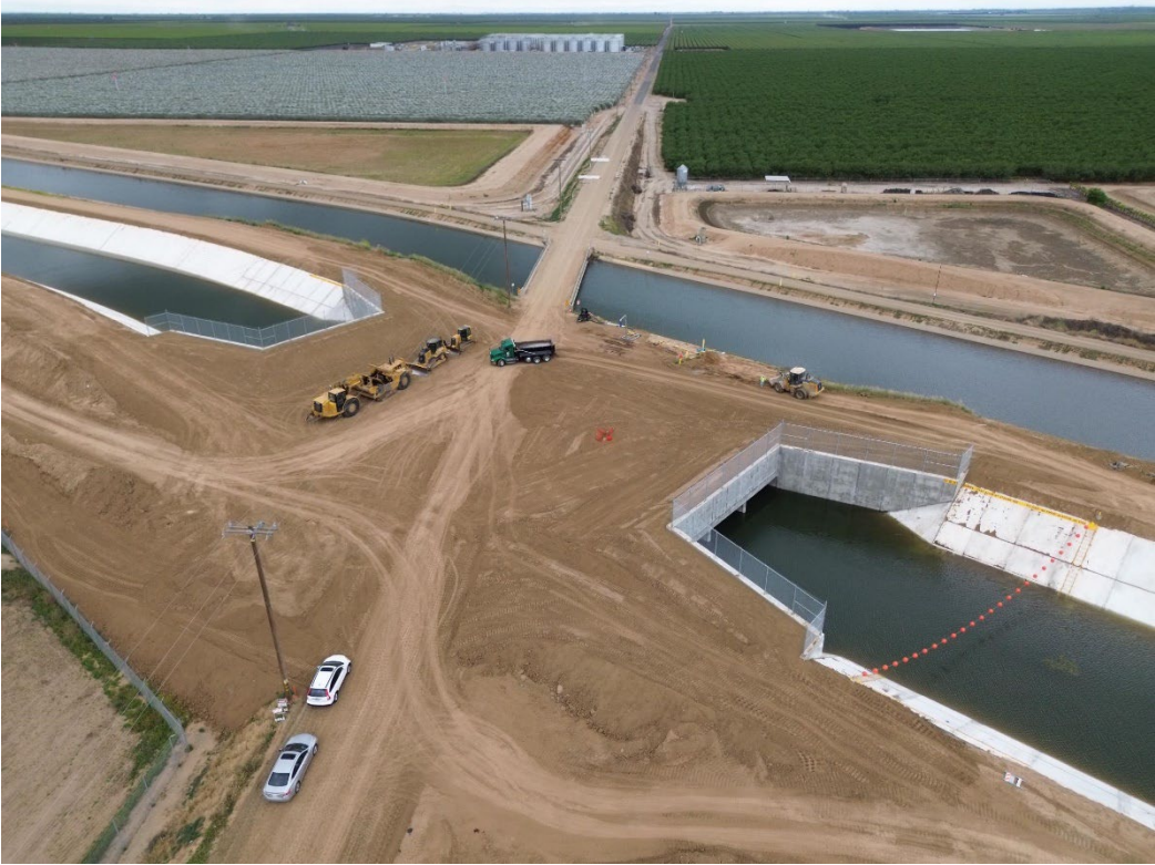
Backfill Completed at Avenue 80 Siphon.
