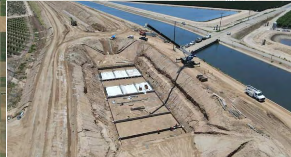
Avenue 80 siphon excavation and foundation slab
