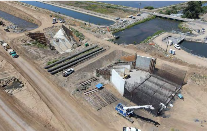
Deer Creek check formwork in progress
