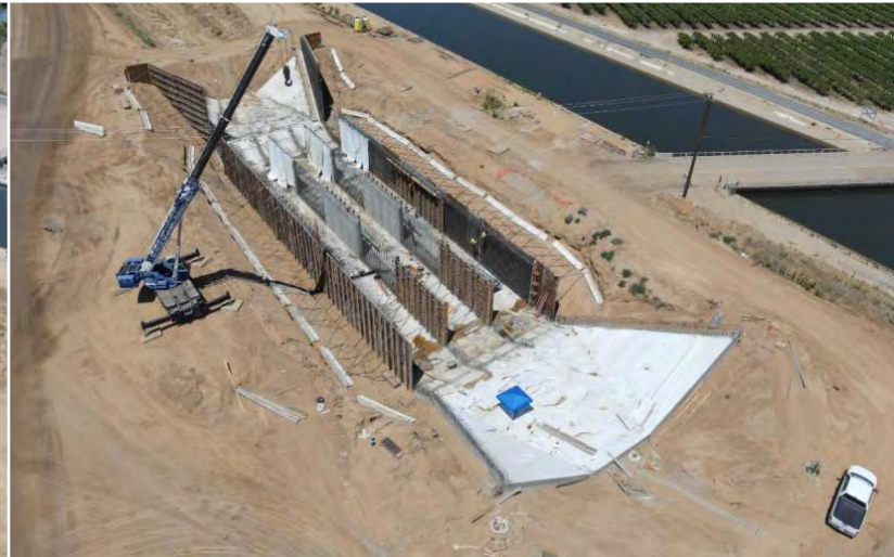
Road 208 siphon wall placement in progress
