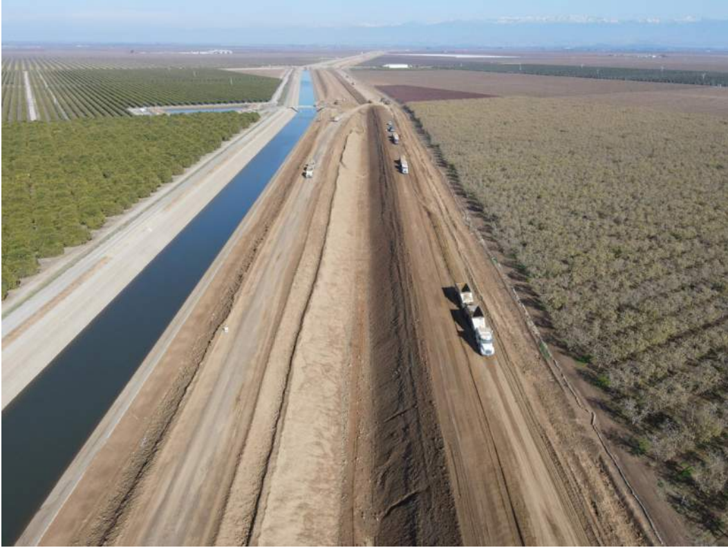
Canal Embankment South of Avenue 88
