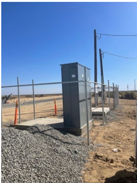
Delano staff install electrical panels at Shafter Check reverse flow pump.
