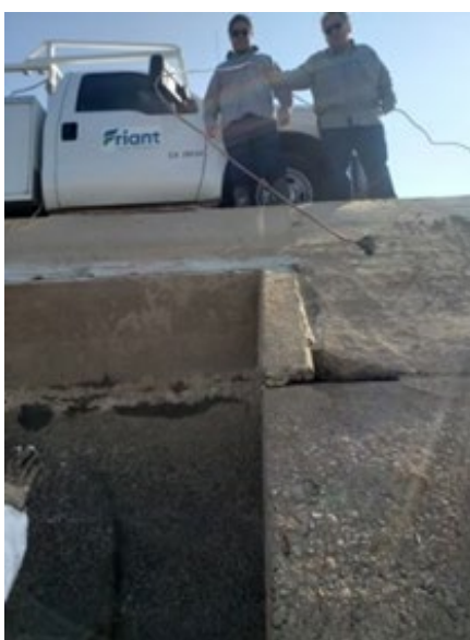
Lindsay staff sealed inlet drains, patched concrete surroundings, and sandbagged the flap valves in the MRCCP area to prevent leakage into the construction area
