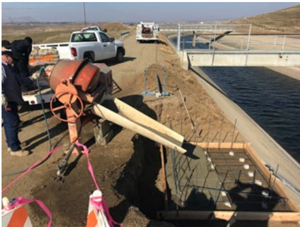
OC staff placing concrete foundation for the measuring bridge.
