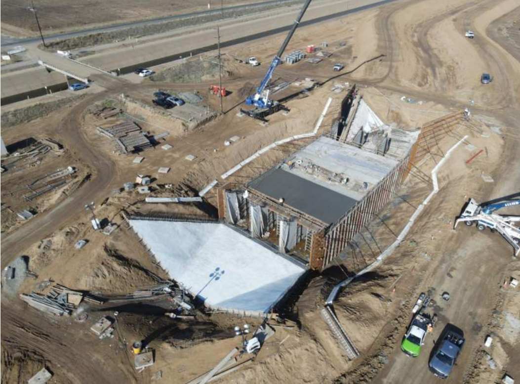
Avenue 112 Siphon Showing Concrete Deck Placement in Progress
