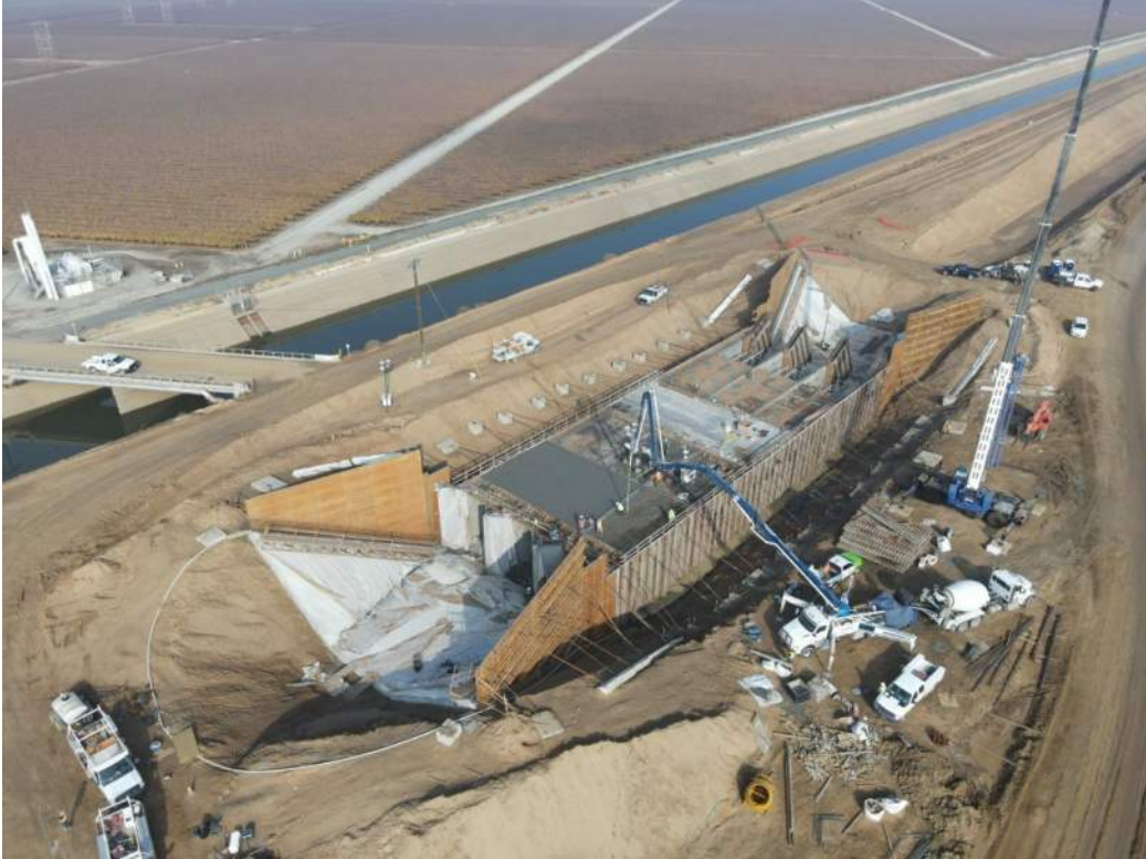
Avenue 88 Siphon Showing Concrete Deck Placement in Progress
