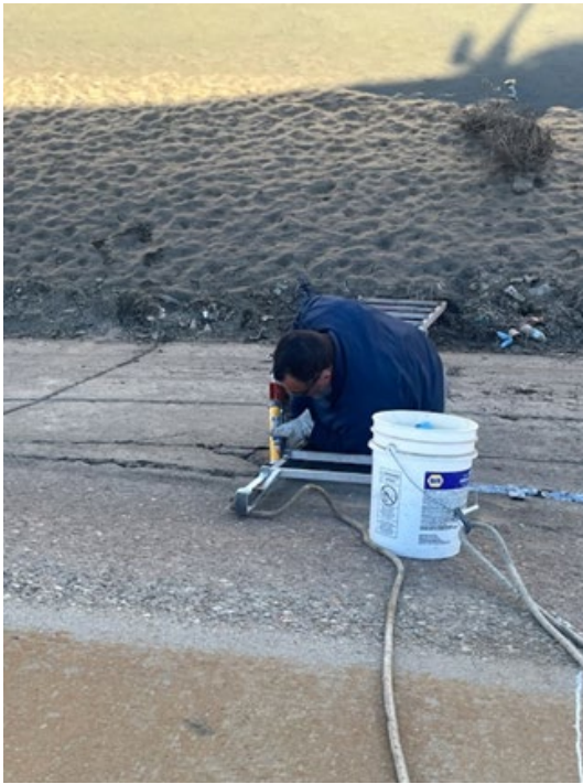
Delano staff-initiated panel replacement and liner sealant repairs, 2.5 panels replaced due to separation and corrosion at MP. 144 and 128
