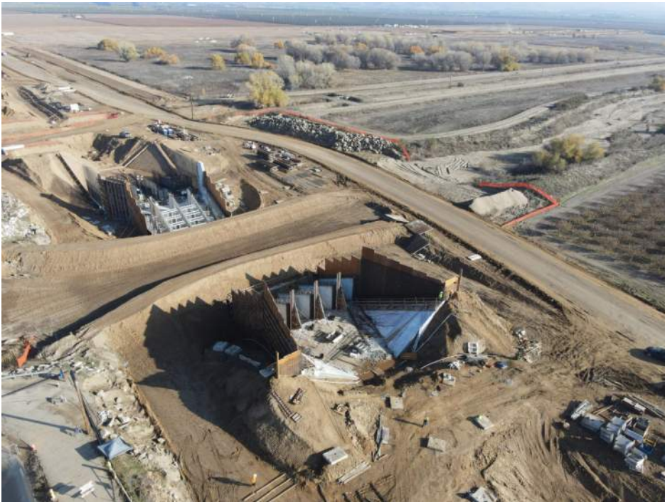
Deer Creek Site showing Temporary Diversion Berms Across Siphon
