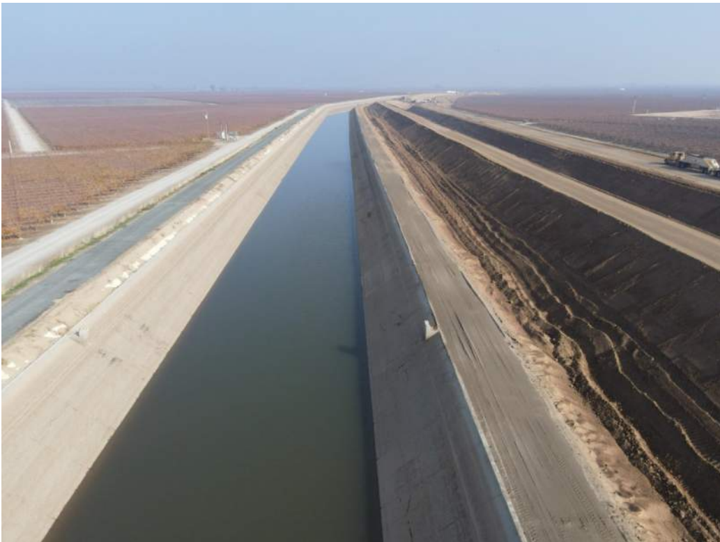
Canal Embankment North of Avenue 88
