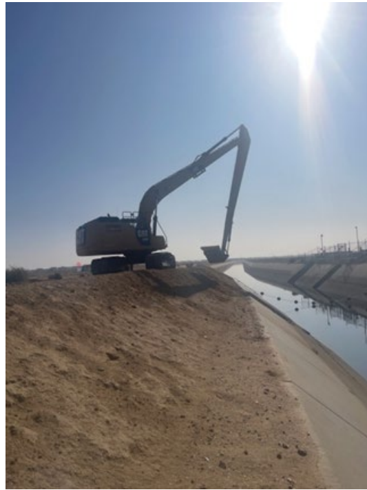
Delano staff-initiated panel replacement and liner sealant repairs, 2.5 panels replaced due to separation and corrosion at MP. 144 and 128
