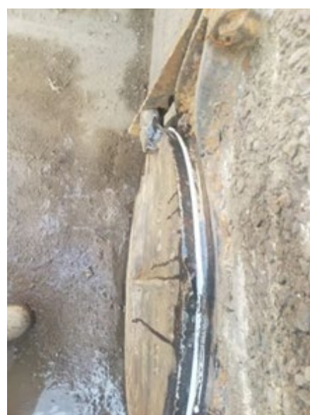
Lindsay staff sealed inlet drains, patched concrete surroundings, and sandbagged the flap valves in the MRCCP area to prevent leakage into the construction area
