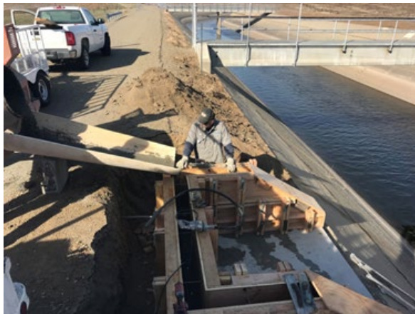
OC staff placing concrete foundation for the measuring bridge.
