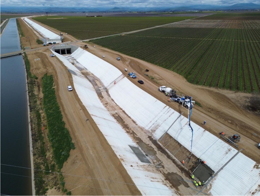
Canal Lining Panel Replacement.
