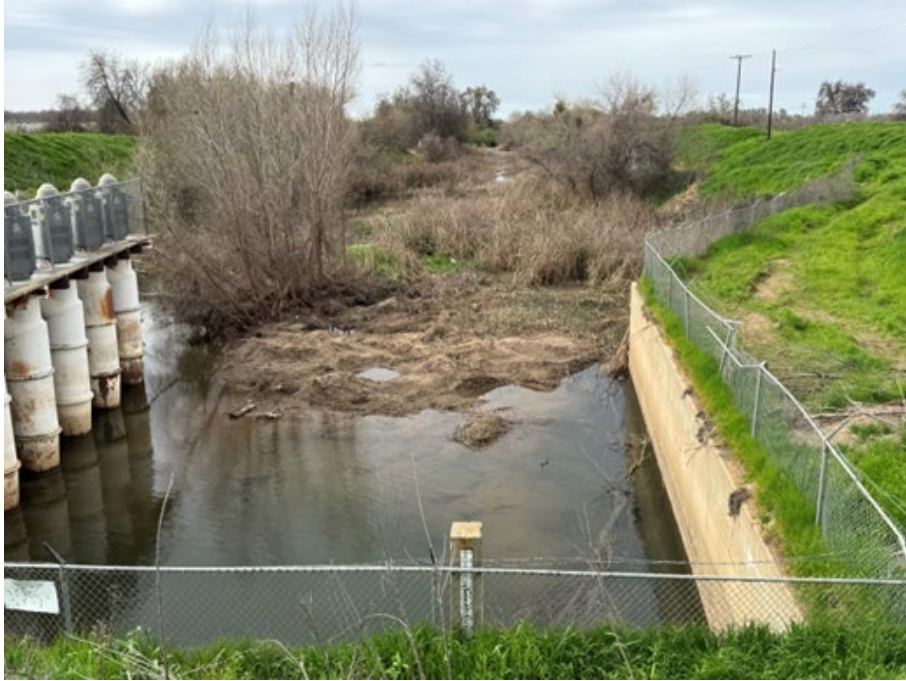
OC staff began desilting project at the St. Johns wasteway.
