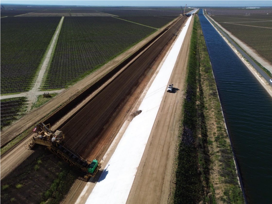
Canal Trimming Completed.
