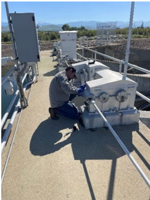
Lindsay staff cleaned and pressure washed motors gearboxes and turnout pedestals on FKC.
