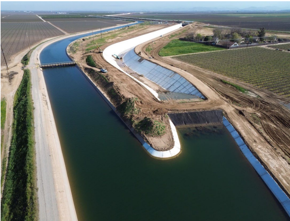
View of the South Tie-in Showing the South Temporary Plug.
