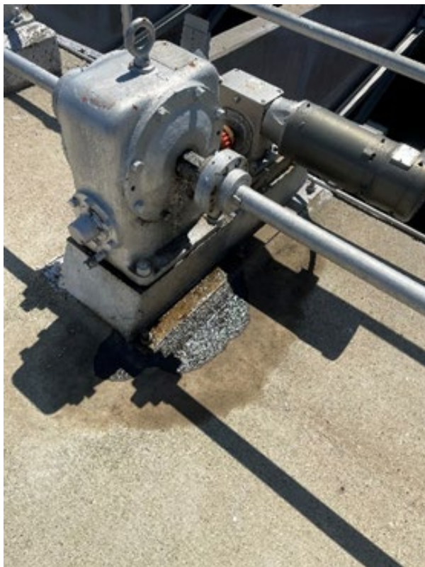
Lindsay staff cleaned and pressure washed motors gearboxes and turnout pedestals on FKC.
