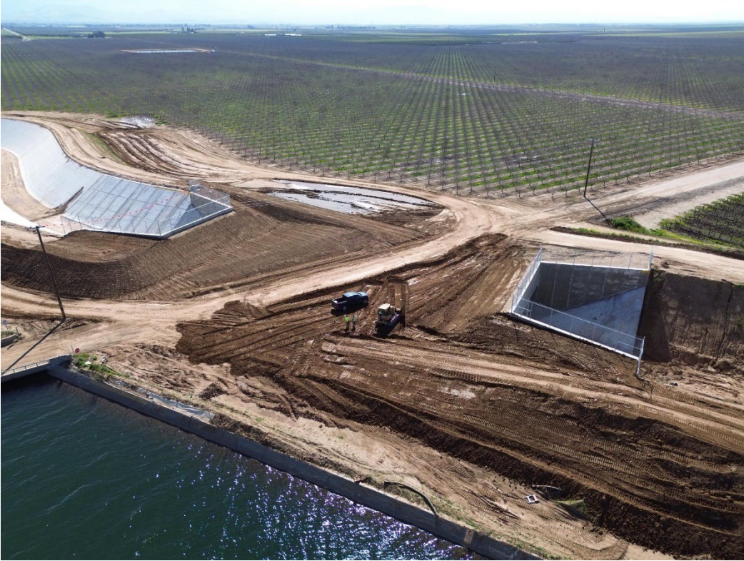
Grading Road 208 and Around the Siphon.
