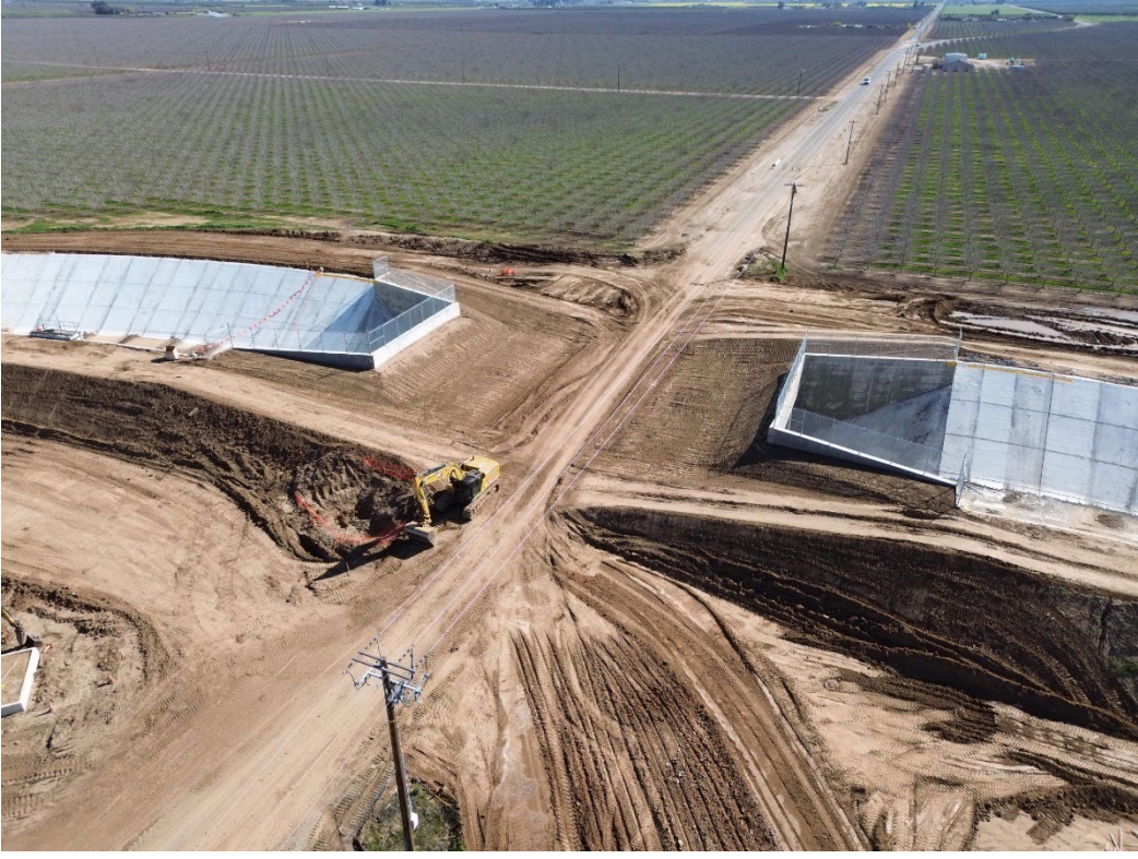
Grading Avenue 95 and Around the Siphon.
