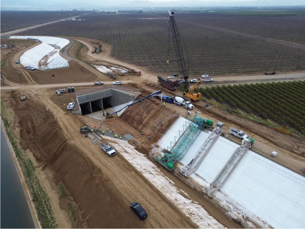
Canal Machine Lining Completed Between Avenue 88 and Road 208.
