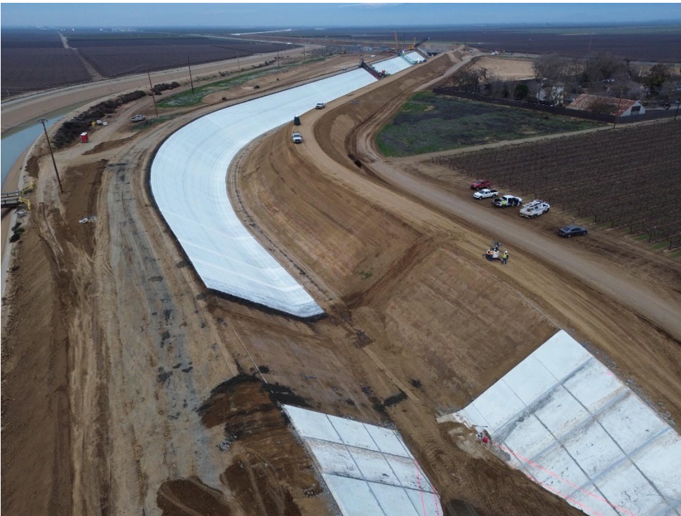
Machine Paving on Southern End of Alignment.
