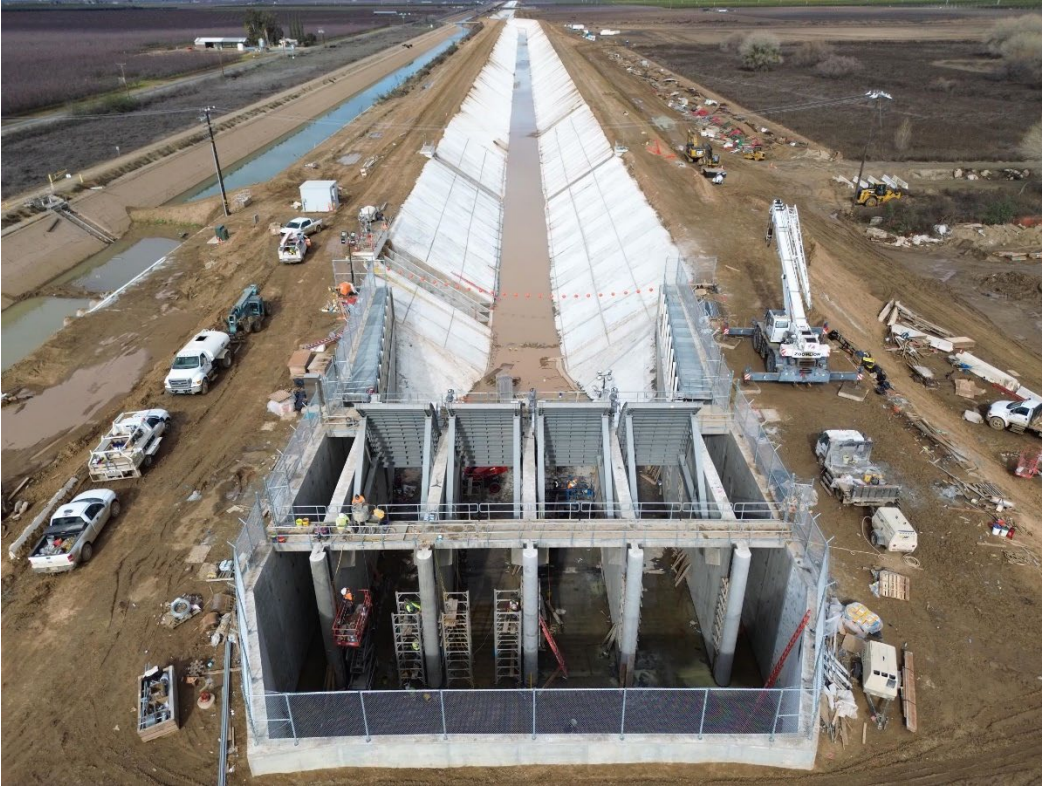
Deer Creek Check Looking Northwards Showing the Radial Gates.
