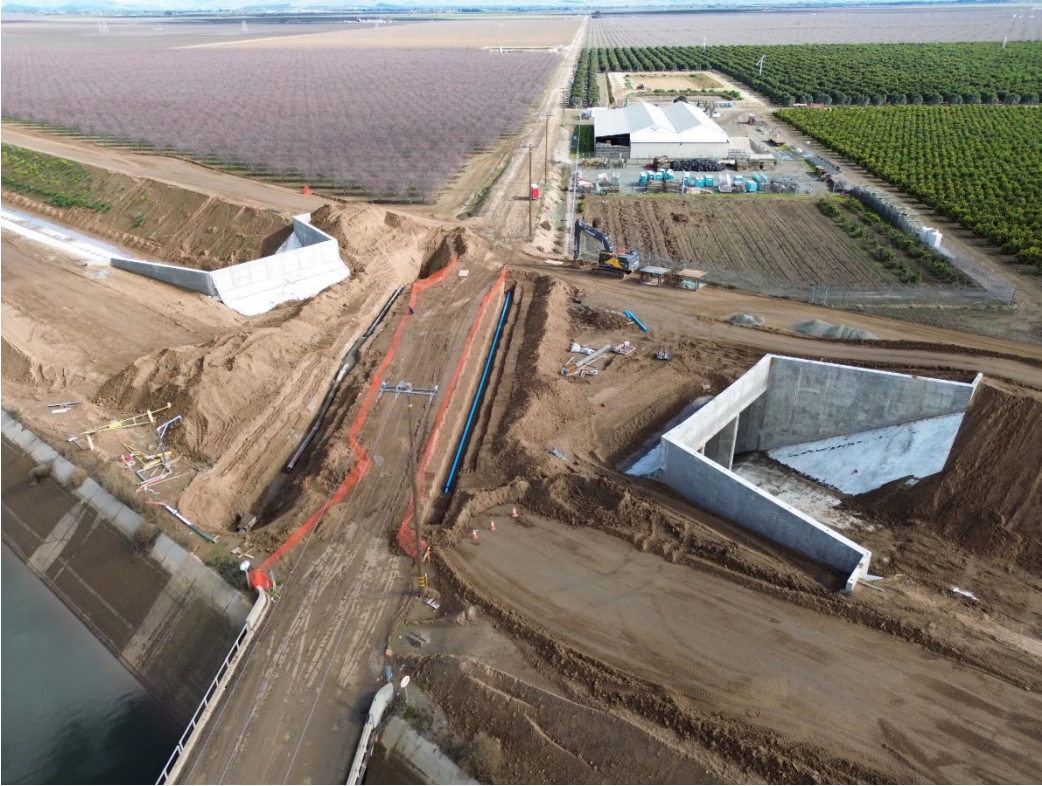
Avenue 80 Siphon with the Irrigation Pipe Installation in Progress.
