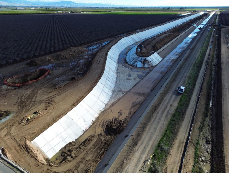
North Canal Tie-in Point Joint Sealing in Progress.
