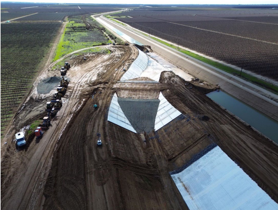
Temporary Earthen Plug at South Tie-in Point.
