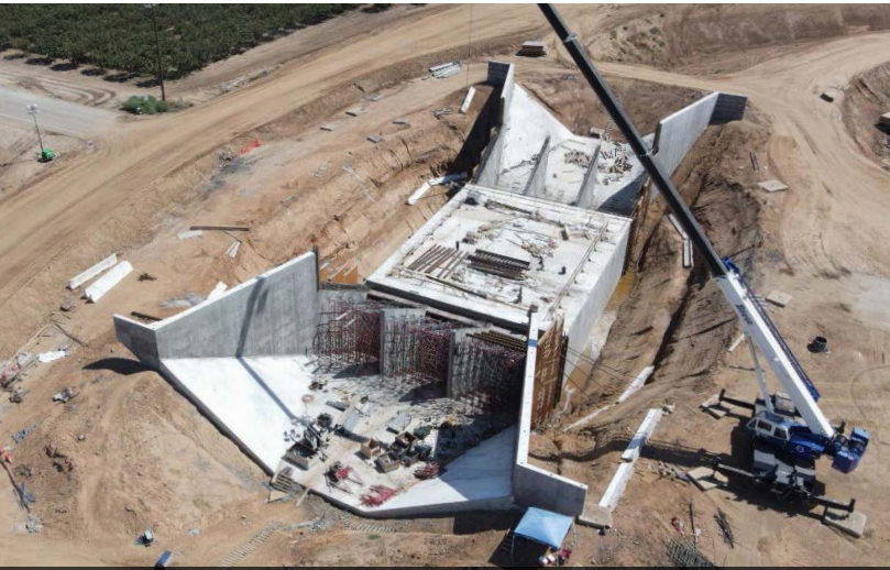
Avenue 95 siphon framework for the sloped deck section in progress
