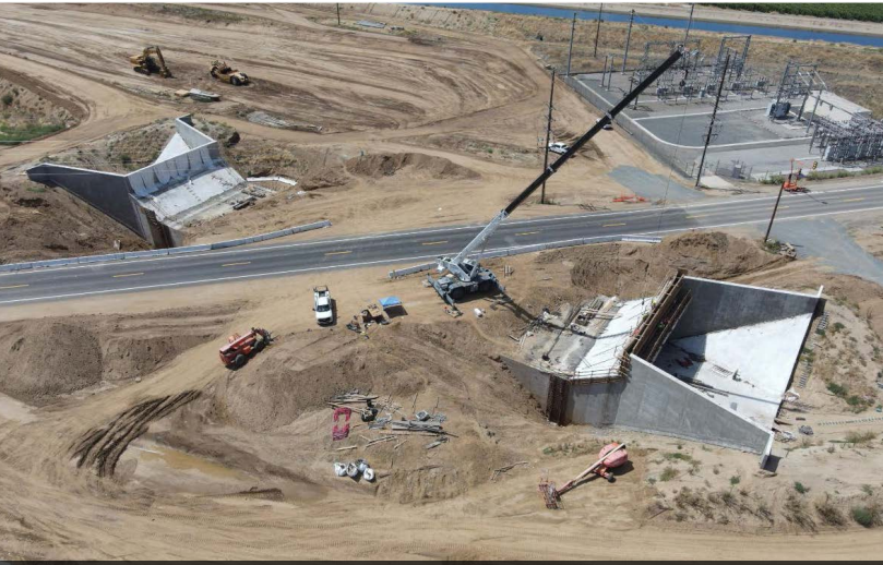
Road 192 siphon concrete structure completed 8/25/23
