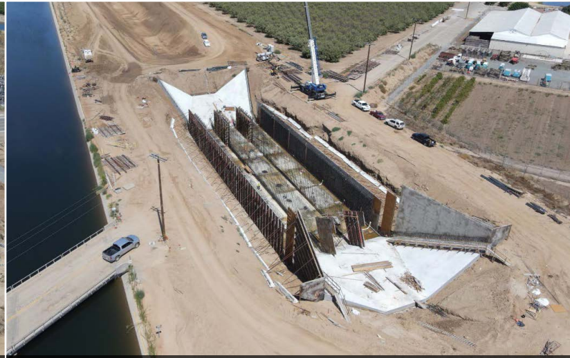
Avenue 80 wall reinforcement and framework in progress
