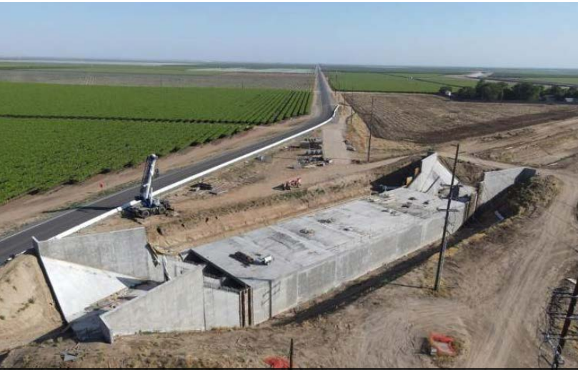
Road 192 Siphon - Falsework Removal in Progress
