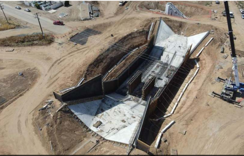
Avenue 95 Siphon Wall Reinforcement / Formwork in Progress
