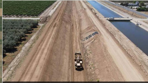
Canal Embankment Final Invert Grading south of Avenue 128
