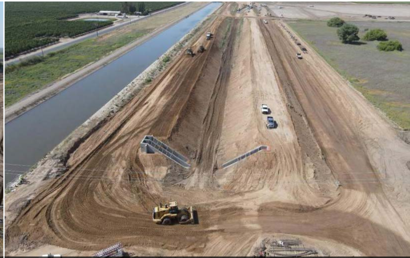
Canal Embankment Construction North of DCTRA Pits and SID-S2 Turnouts
