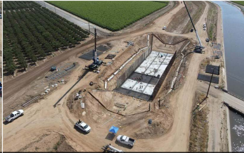
Road 208 Siphon Invert Slab Construction in Progress
