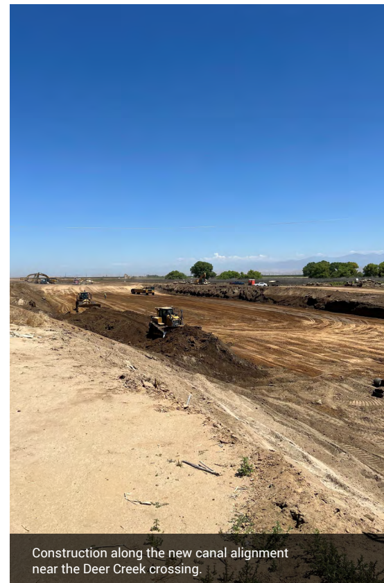
Excavator and scraper working on excavating the existing canal embankment and backfilling the new embankment.
