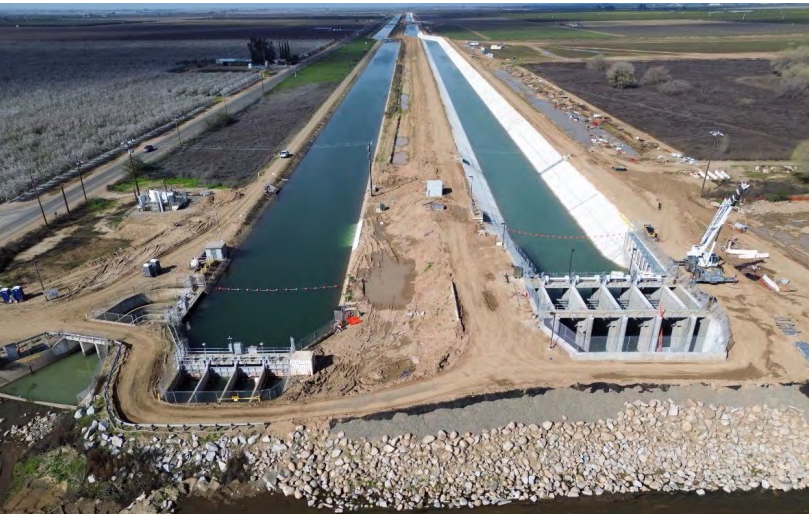
Existing and new Deer Creek Check Structures looking northwards
