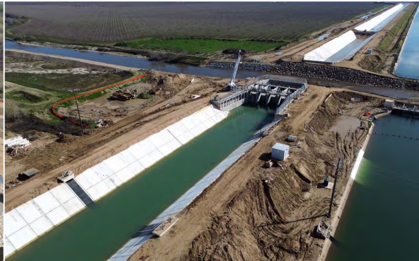
Deer Creek Wasteway and Check Structure and DCTRA and SID-S2 turnouts
