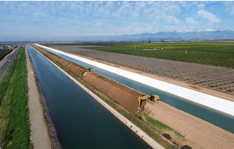
Earthen freeboard placement and compaction
