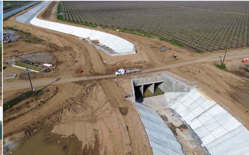
Siphon leak test in progress at Ave. 95
