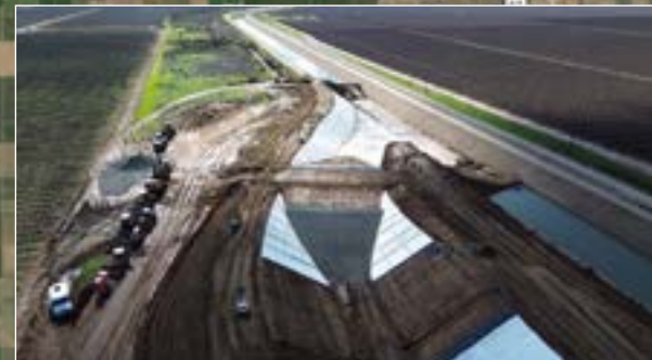
Temporary earthen plug at south tie-in point
