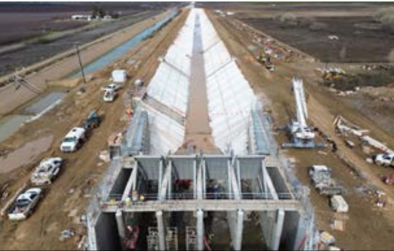
Deer Creek check looking northwards showing the radial gates
