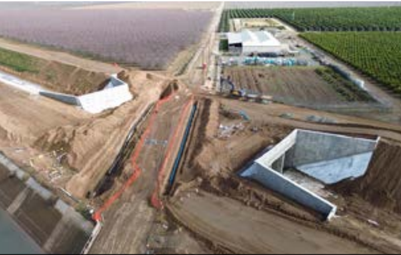
Ave 80 siphon with the irrigation pipe installation in progress
