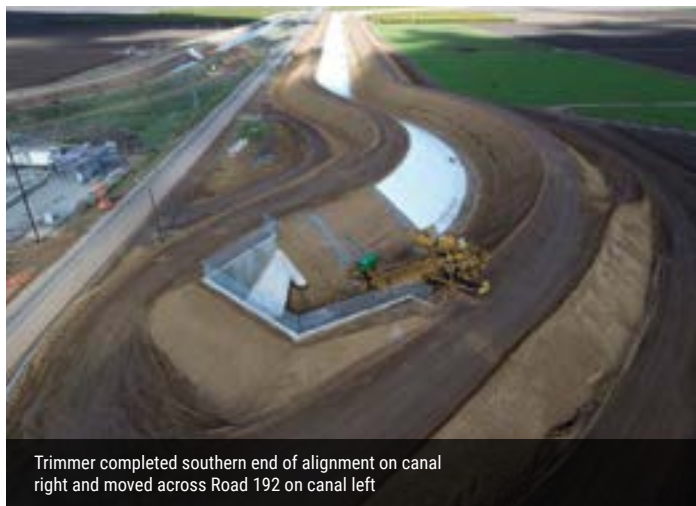
Machine paving on souther end of alignment
