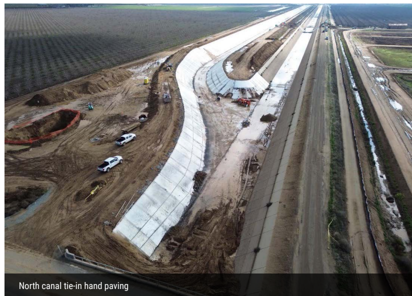
Canal paving on Canal Right south of Avenue 80
