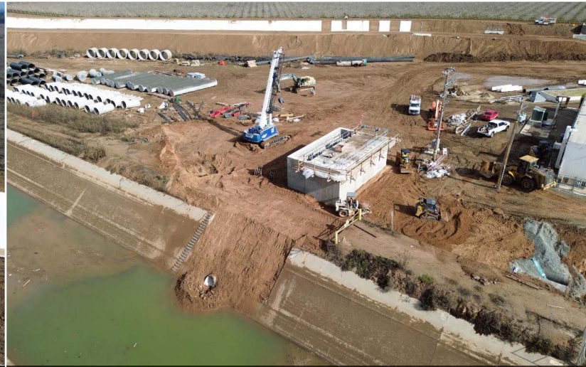
Terra Bella ID weir box and outfall pipe installation
