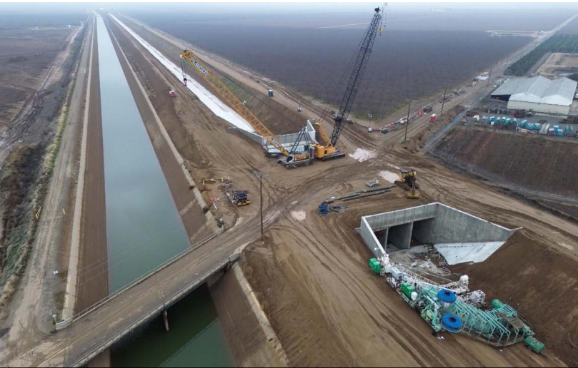
Avenue 80 siphon falsework removal in progress and structural backfill partially complete
