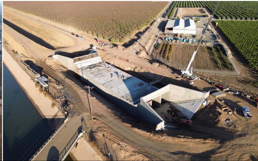
Avenue 88 siphon formwork and falsework removal
