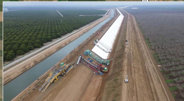
Canal paving on Canal Right south of Avenue 80
