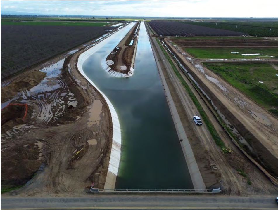
North Canal Tie-In At Avenue 136.
