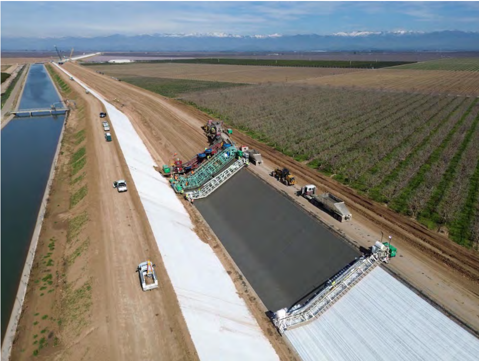
Canal Machine Paving Near Avenue 74 Bridge.
