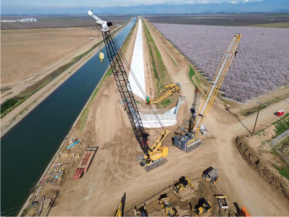
Canal Trimming Equipment North of Avenue 80.
