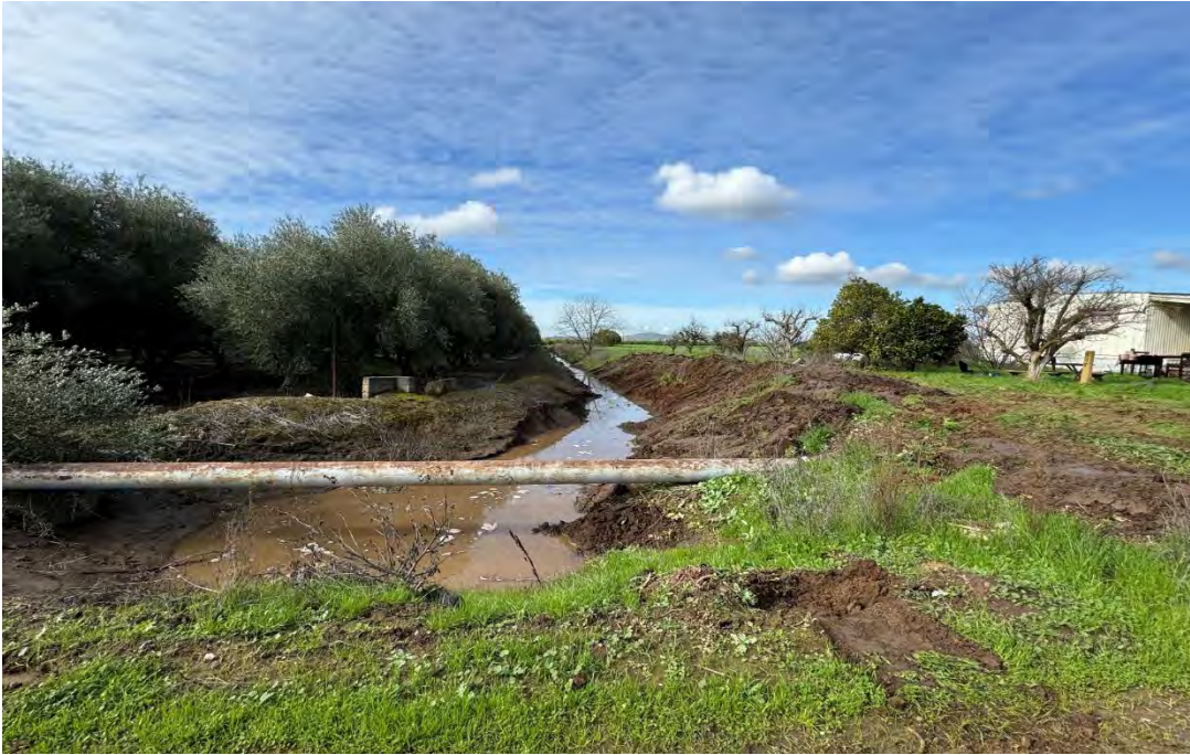
Orange Cove staff cleaning a cross-drain to help prevent local flooding.
