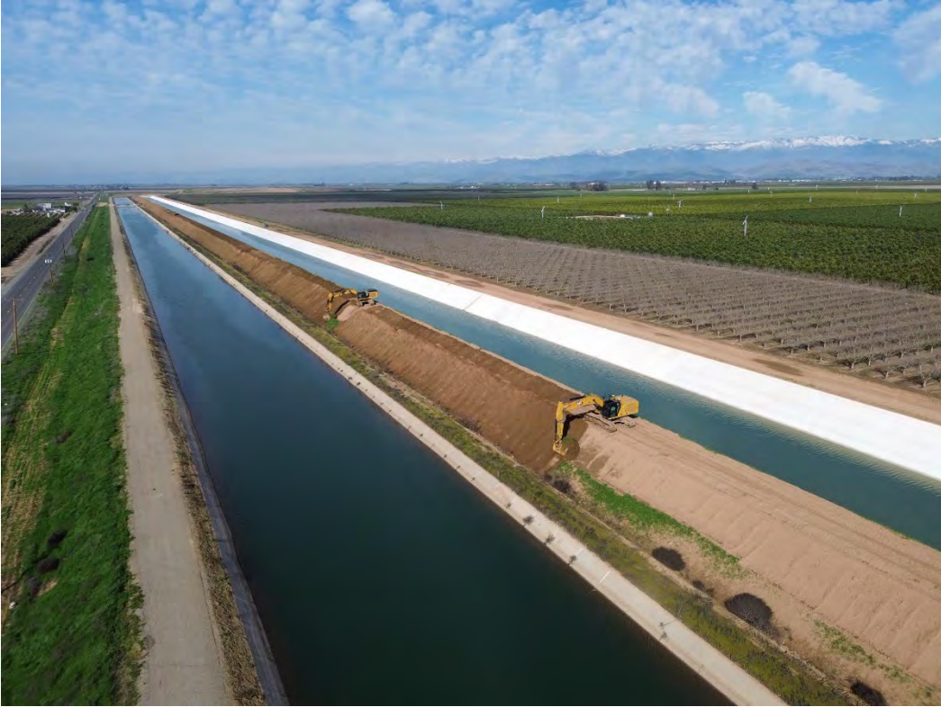
Earthen Freeboard Placement And Compaction.
