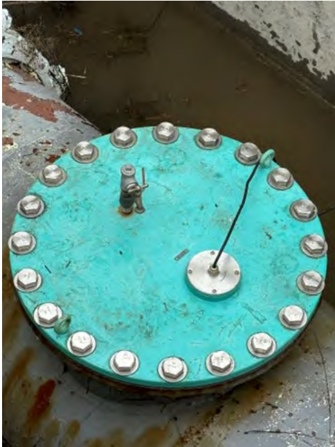
Kern Tulare #4 Meter leak repair
