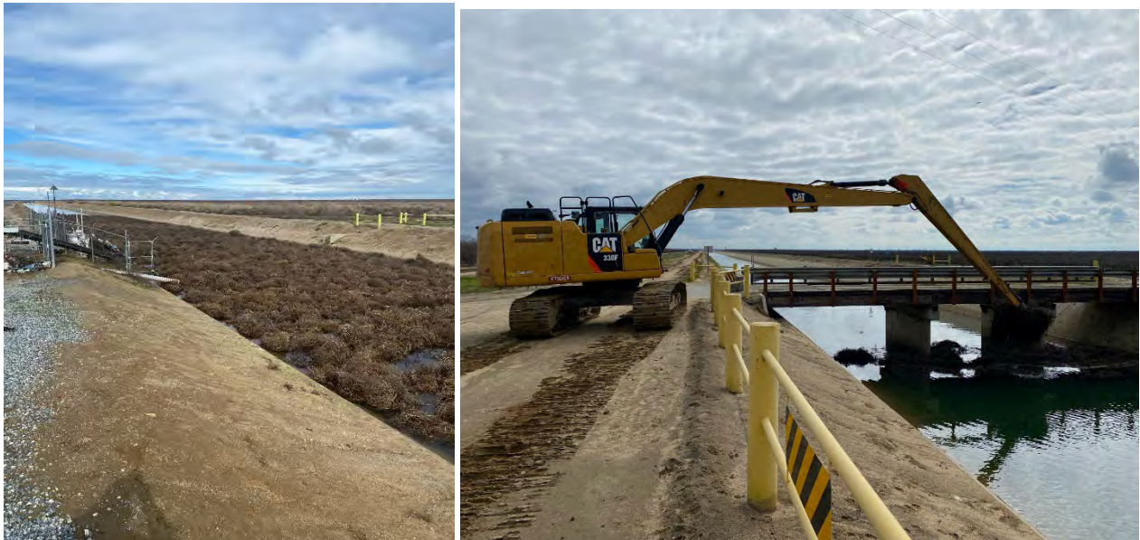
Orange Cove staff removing tumbleweeds and debris with excavator.
