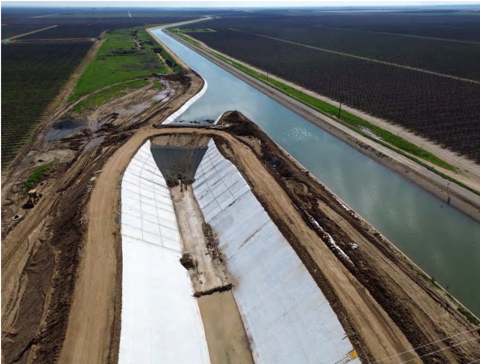
South Canal Tie-in Hand Paving Completed.
