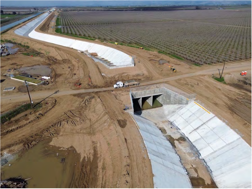
Siphon Leak Test In Progress At Avenue 95.
