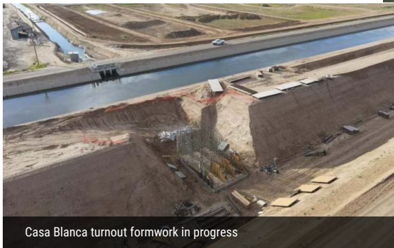
Road 192 siphon structure
