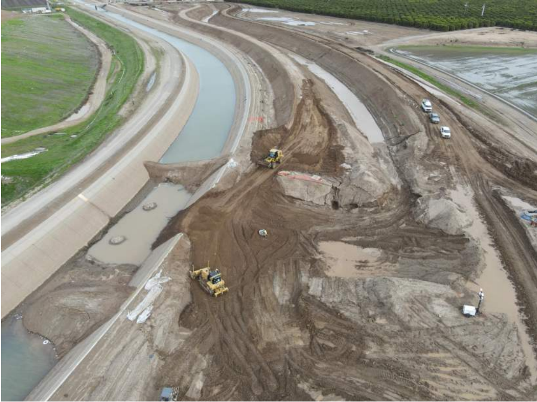
South of Avenue 128 - 5x4 drainage extension box backfilling in progress - 01/13/23
