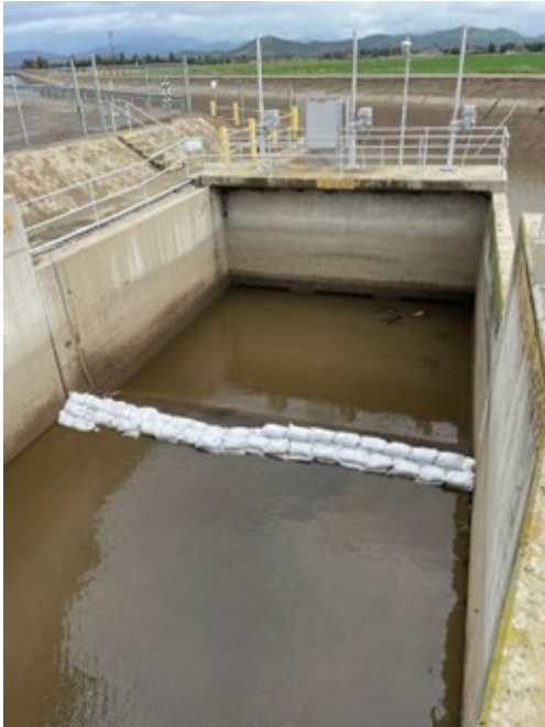
Lindsay staff placed sandbags and pumps at Tule River wasteway to stop water from entering the canal which was required to be isolated for construction.
