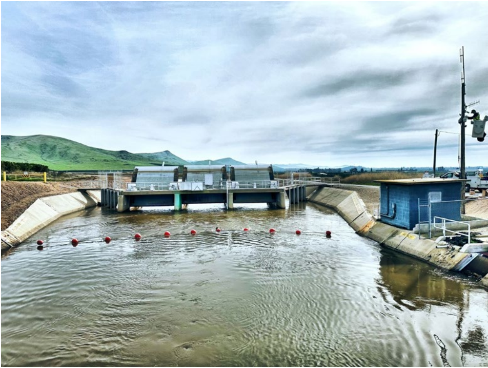
Camera Installation at Rocky Hill
