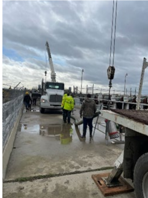
Lindsay staff placed sandbags and pumps at Tule River wasteway to stop water from entering the canal which was required to be isolated for construction.
