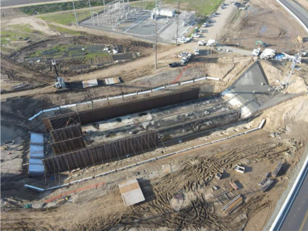
Road 192 siphon concrete slab placement
