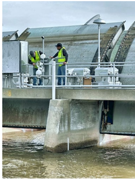
Camera install on the Rocky Hill Check structure
