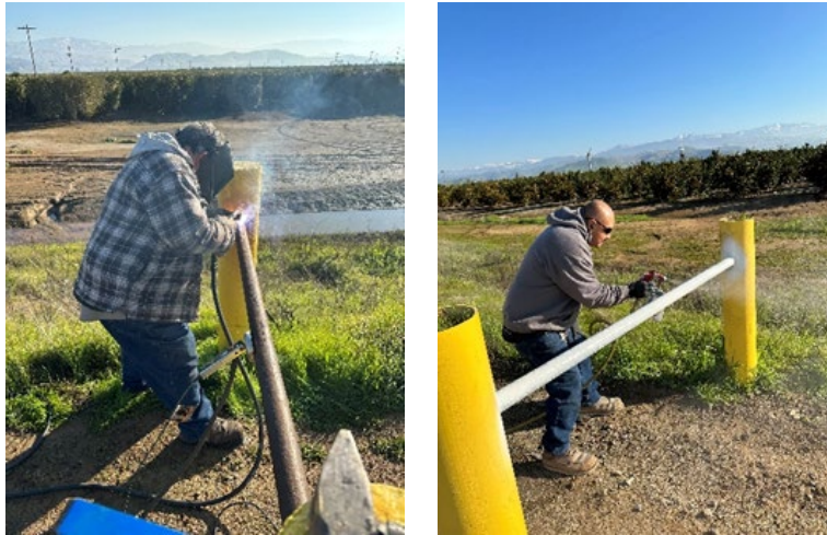
Lindsay maintenance staff repaired and painted guardrails.
