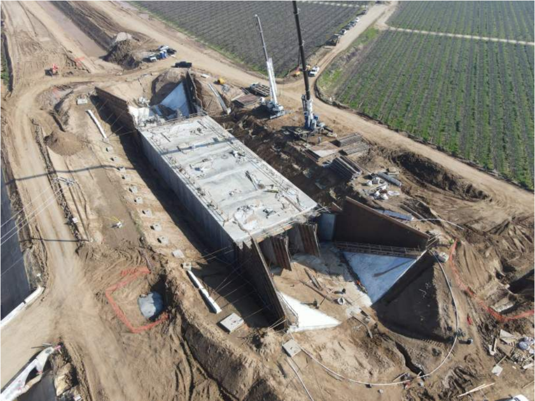
Avenue 88 siphon transition wall reinforcement installation in progress
