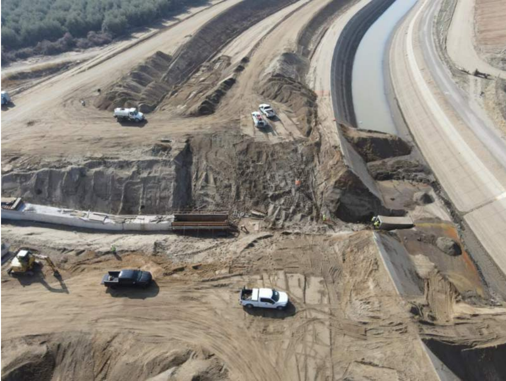
Drainage Box Tie-in During Outage
