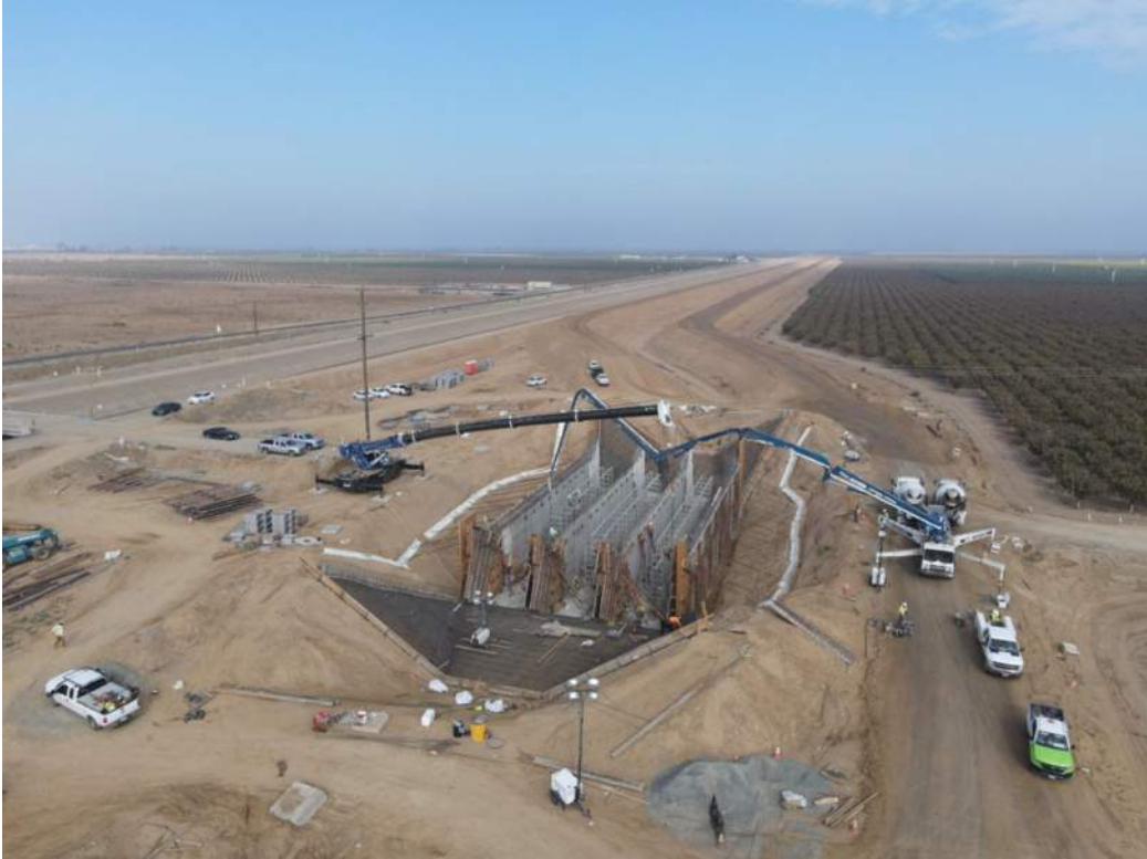
Avenue 112 Siphon – Concrete Wall Placement In Progress
