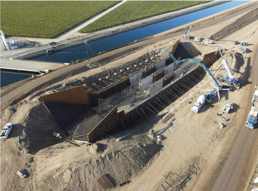
Avenue 88 Siphon – Wall Concrete Placement In Progress
