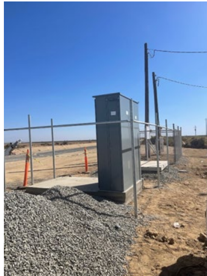
Delano staff installs electrical panels at the Shafter Check
