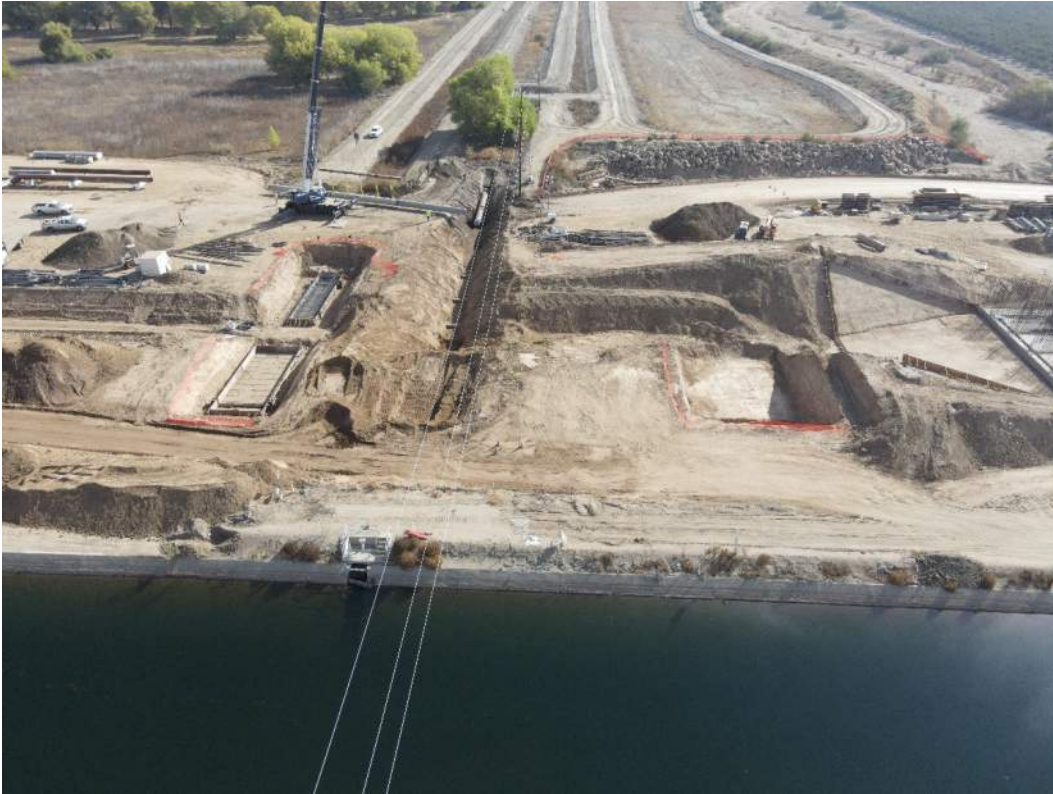
DCTRA Pits, SID-S2, Deer Creek Wasteway Turnouts Area
