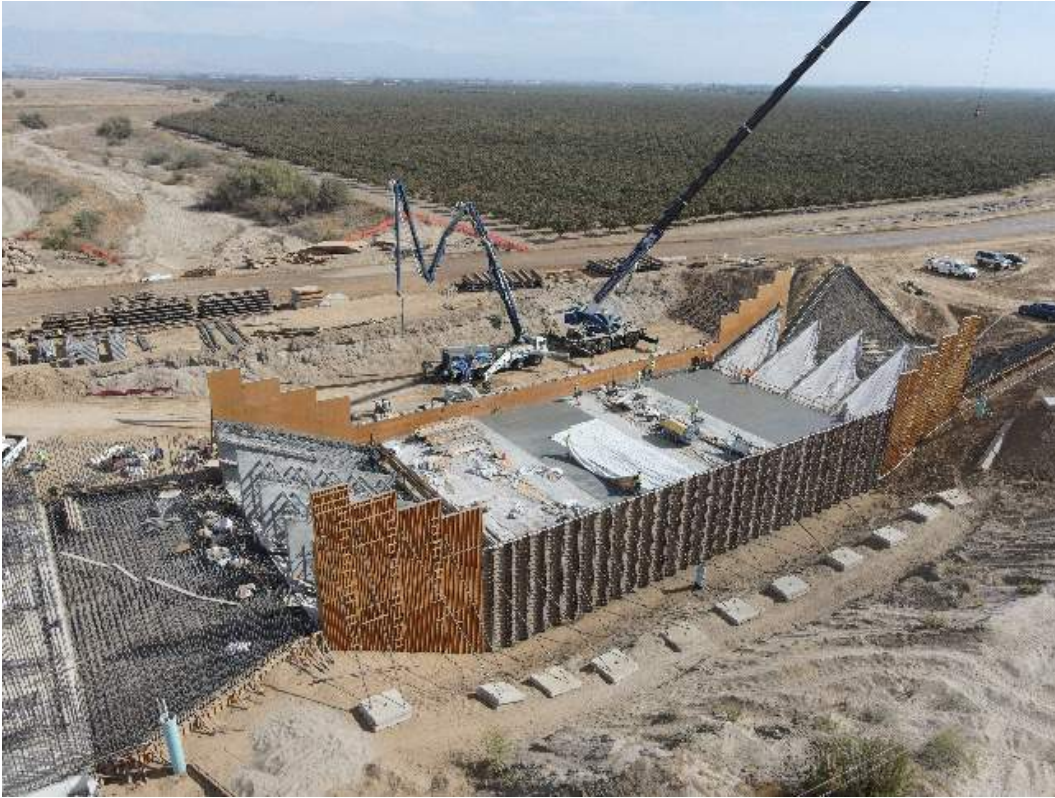
Deer Creek Siphon – Concrete Deck Placement
