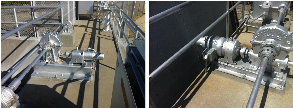
View of Similar Conditions
