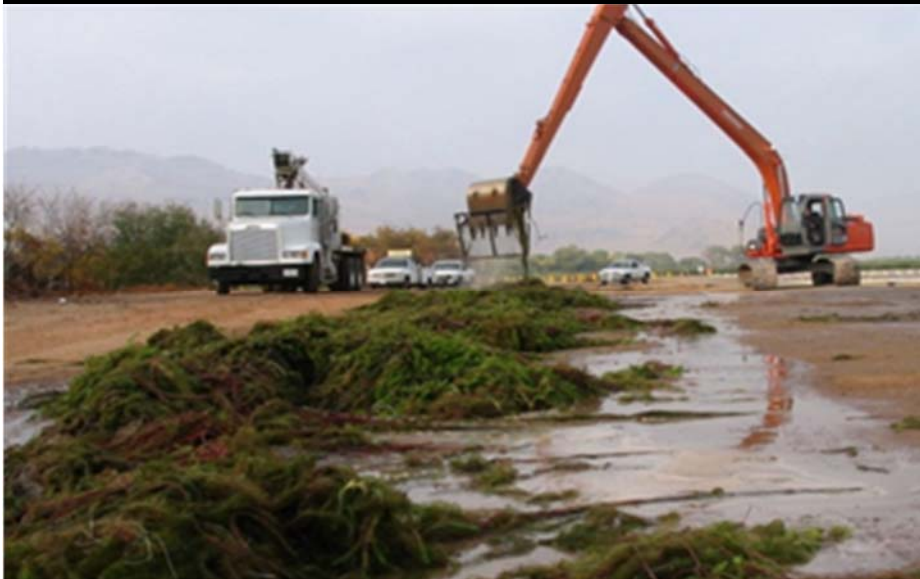
Authority staff removing milfoil from canal prism.
