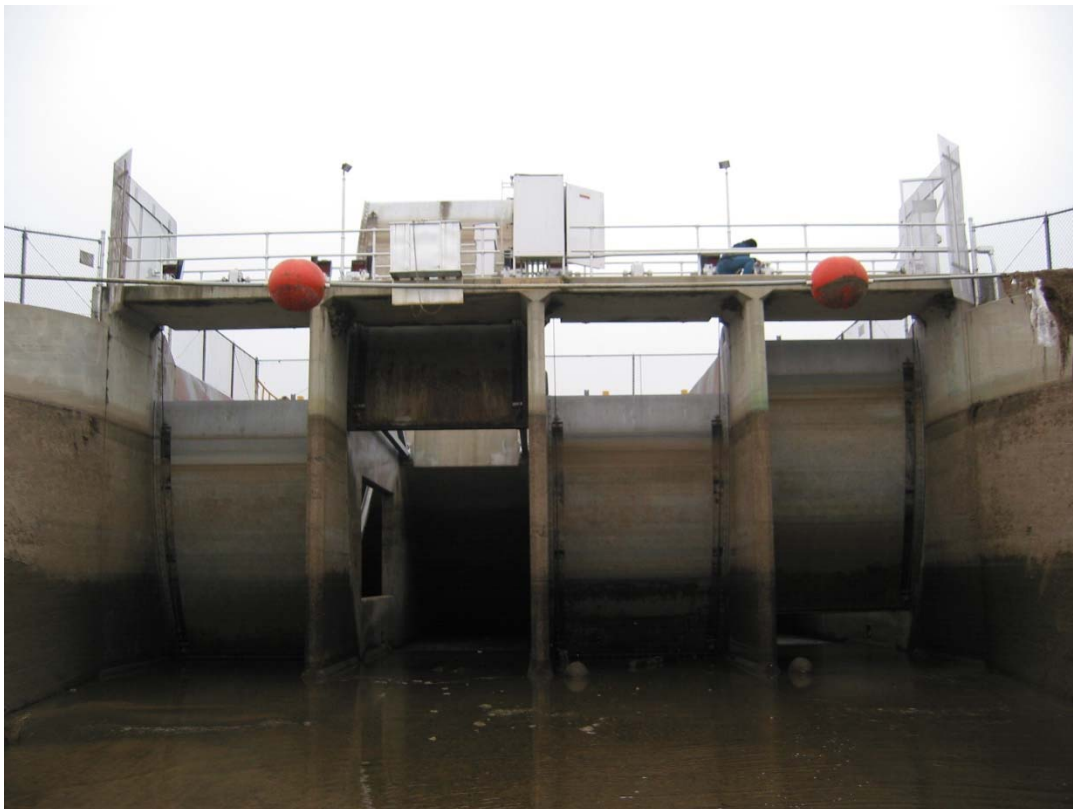
View of Tule River Check Structure
