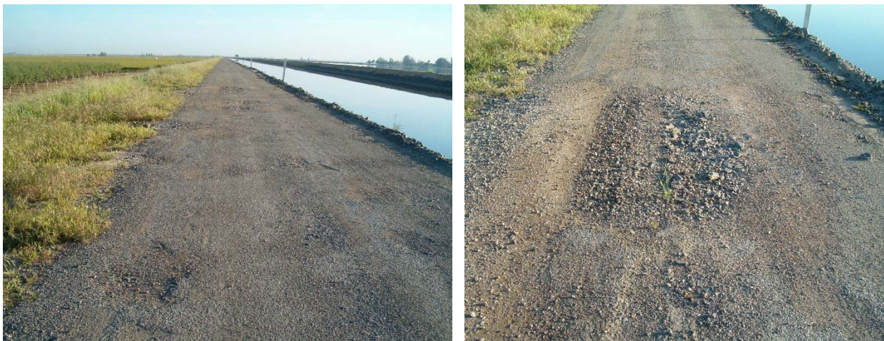
Photo of Existing Conditions
