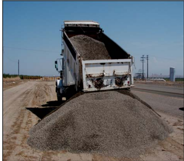
Authority staff placing chip seal stock at project site.
