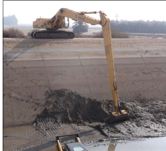
Maintenance staff removing debris from canal prism during dewatering.
