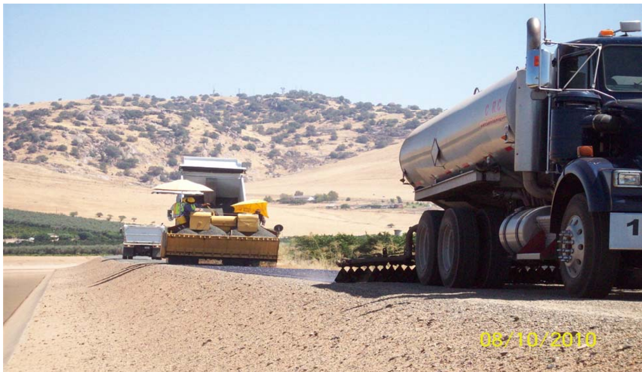
Authority staff placing chip seal along operational roadway.
