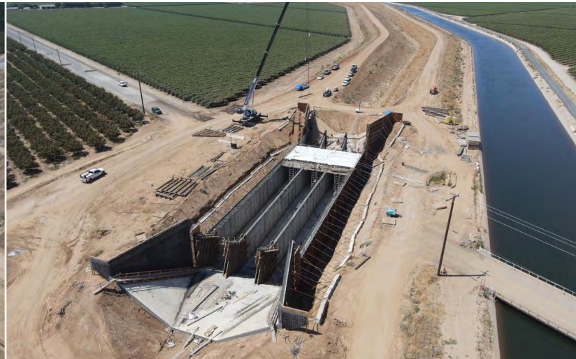
Road 208 siphon - transition wall and deck for the flat section in progress
