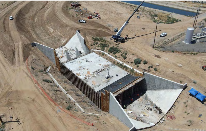
Avenue 128 siphon - sloped deck reinforcement and falsework in progress
