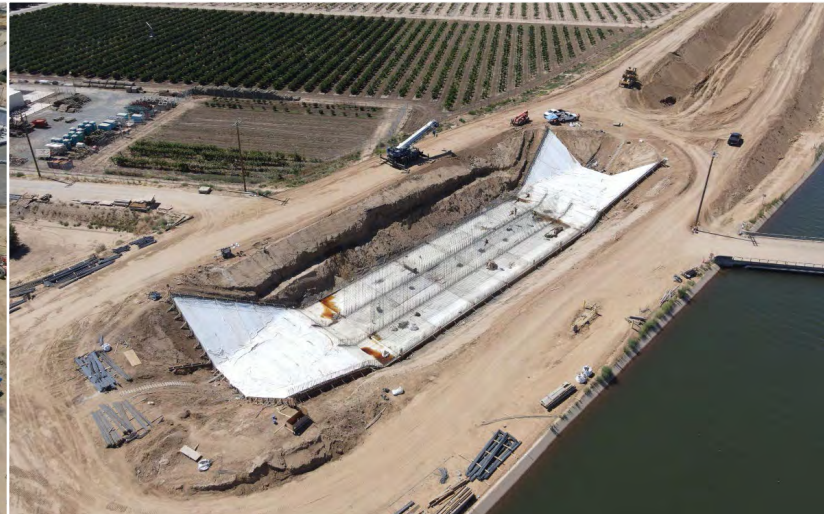
Avenue 80 siphon - slabs curing and wall reinforcement in progress
