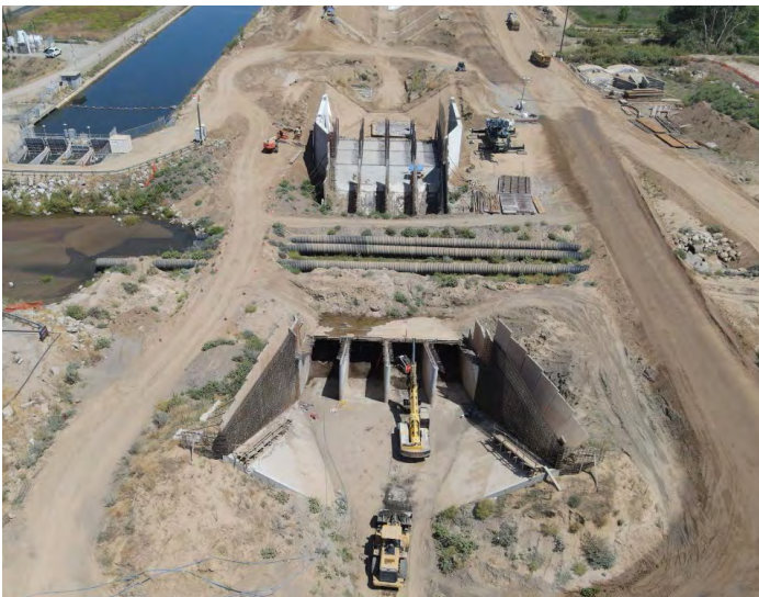
Deer Creek siphon cleanup in progress
