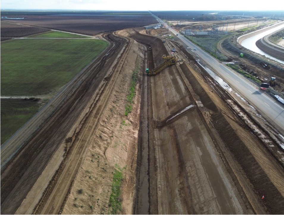
Canal Trimming on Canal Right South of Avenue 80.
