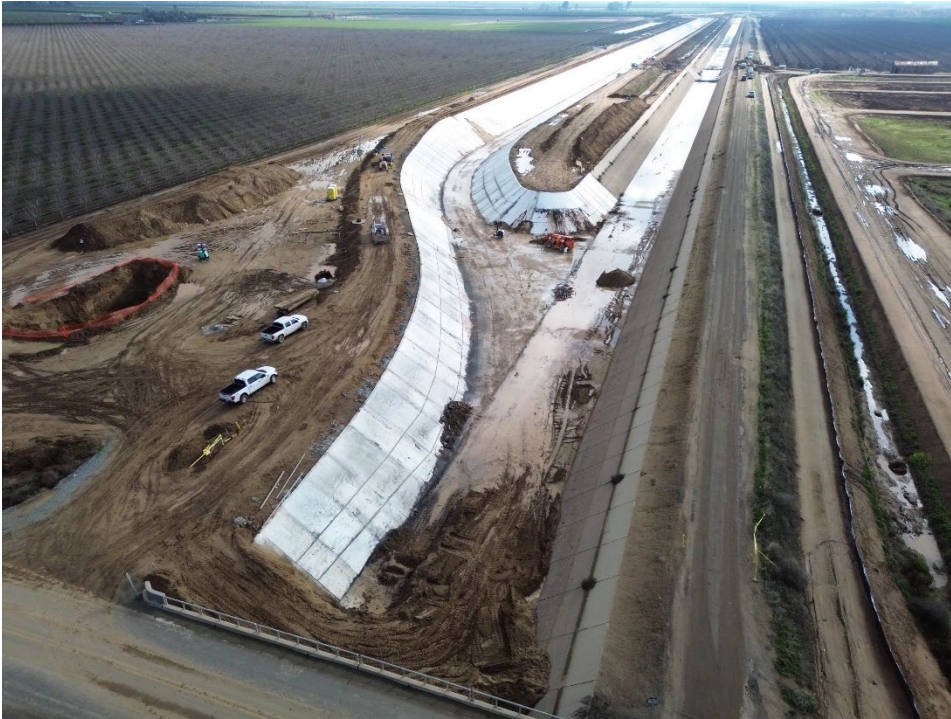
North Canal Tie-in Hand Paving
