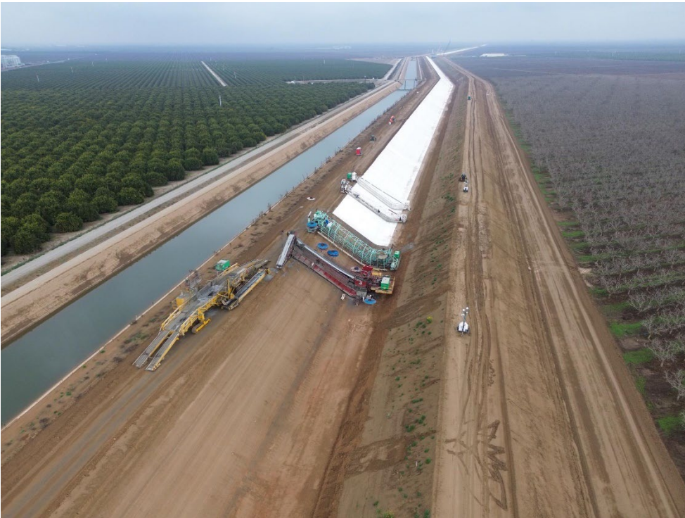
Canal Paving on Canal Right South of Avenue 80.
