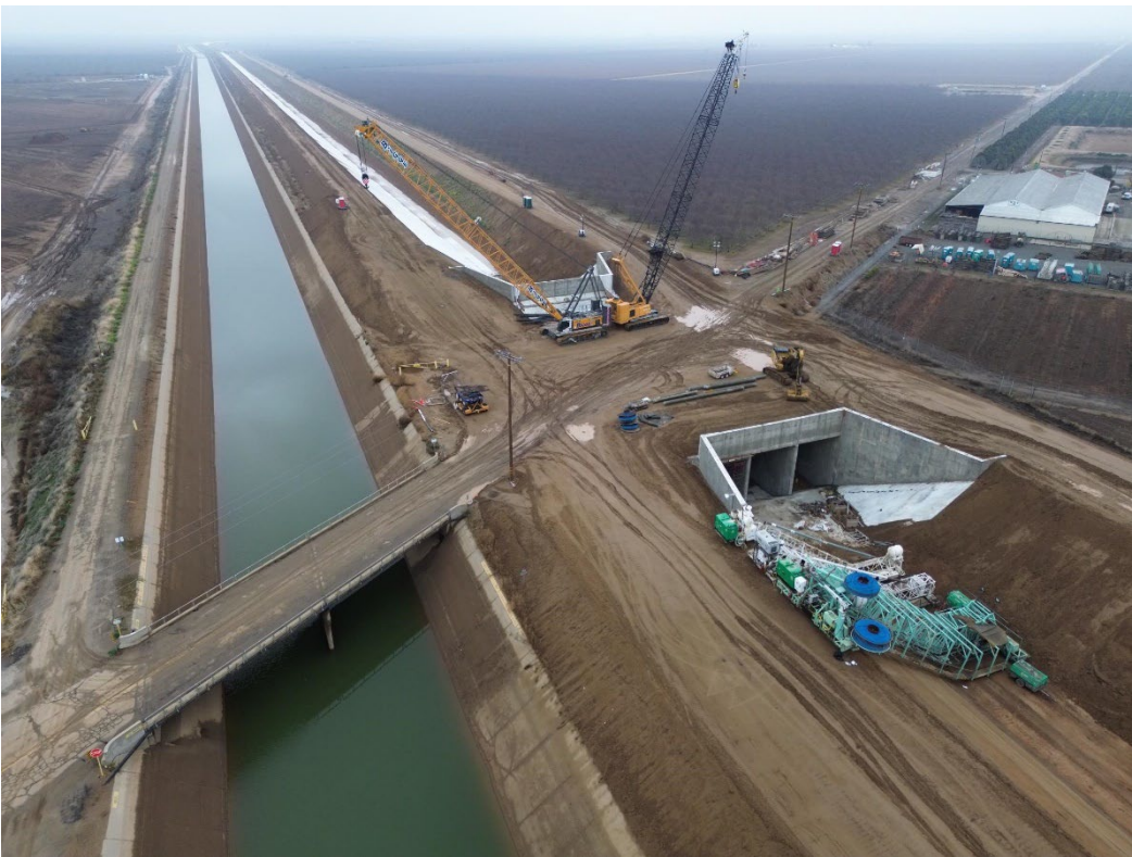
Avenue 80 Siphon Falsework Removal in Progress and Structural Backfill Partially Complete.
