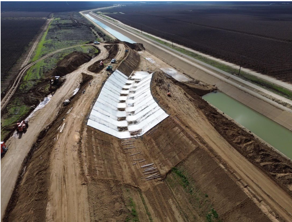
South Canal Tie-in Panel Placement in Progress
