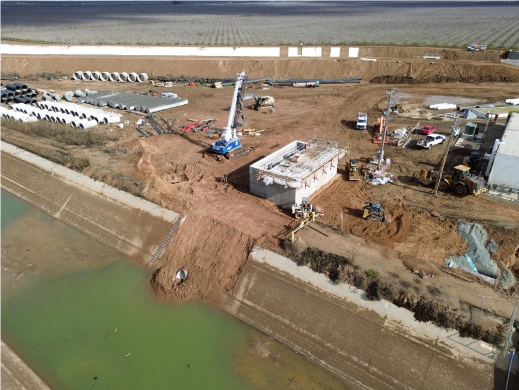
Terra Bella ID Weir Box and Outfall Pipe Installation.
