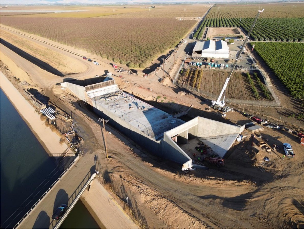
Avenue 88 Siphon Formwork and Falsework Removal.
