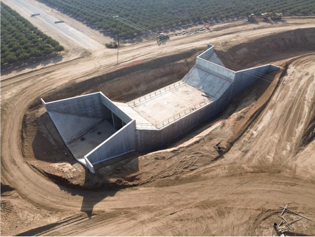
Avenue 95 Siphon south transition backfill being placed.
