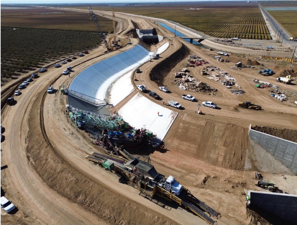
Canal lining in progress south of Terra Bella Avenue to Road 208.
