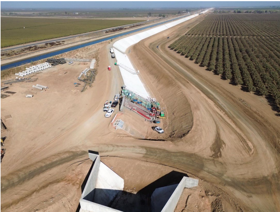
Canal lining completed between Deer Creek Check and Terra Bella Avenue.
