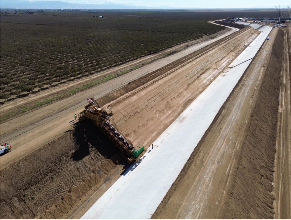
Trimming canal left back towards Deer Creek.
