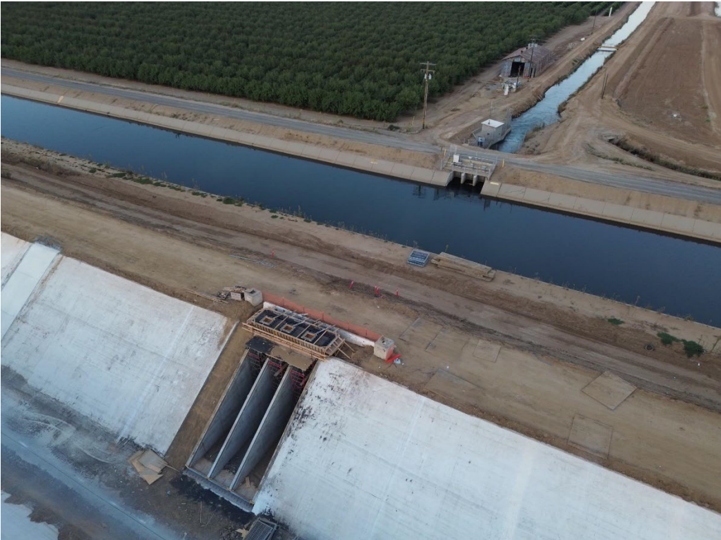
Casa Blanca Turnout top wall and deck were completed.
