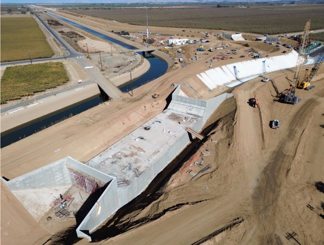
Road 208 Siphon was completed.
